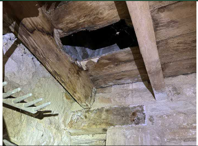
Photograph 8 – Example access between first and ground floors
