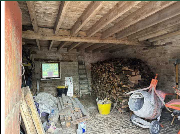
Photograph 7 – Western ground floor room
