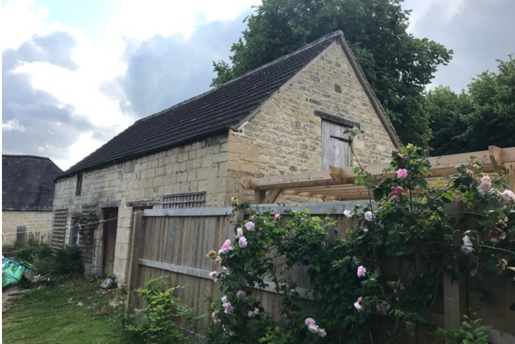
EXISTING BARN VIEWED FROM THE WEST
