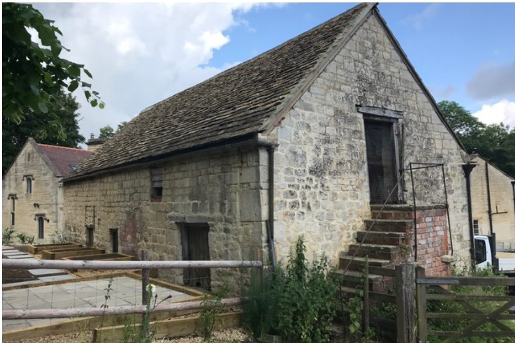
EXISTING BARN VIEWED FROM THE EAST
