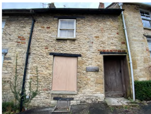
Figure 5: Front elevation of Old Beams
