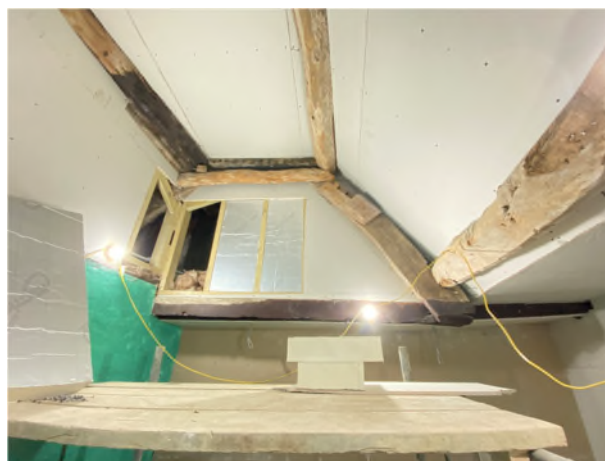
Figure 10: Truncated truss on the first floor
