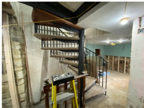
Figure 9: Spiral staircase to the right of the stone chimney breast
