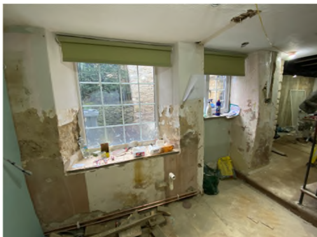
Figure 13: Window openings on the ground floor of Phase 2
