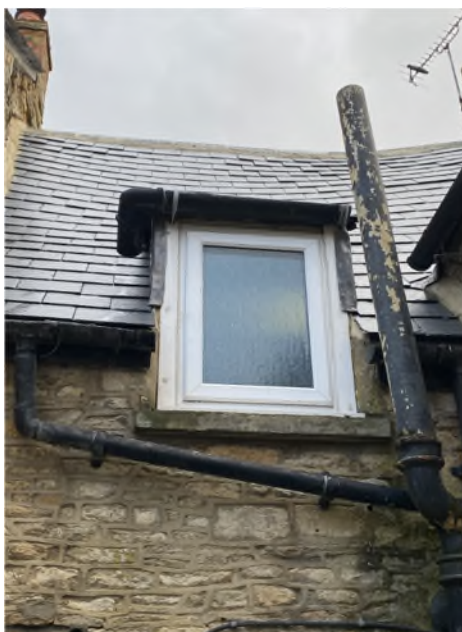
Figure 16: Dormer with a upvc double glazed window on the rear elevation of Phase 1
