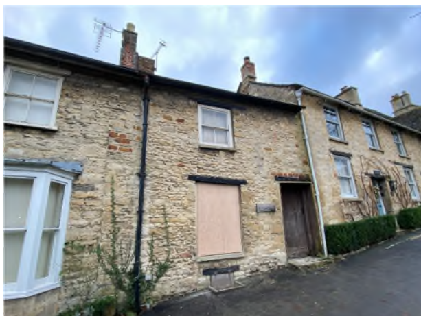
Figure 1: Front elevation of Old Beams
