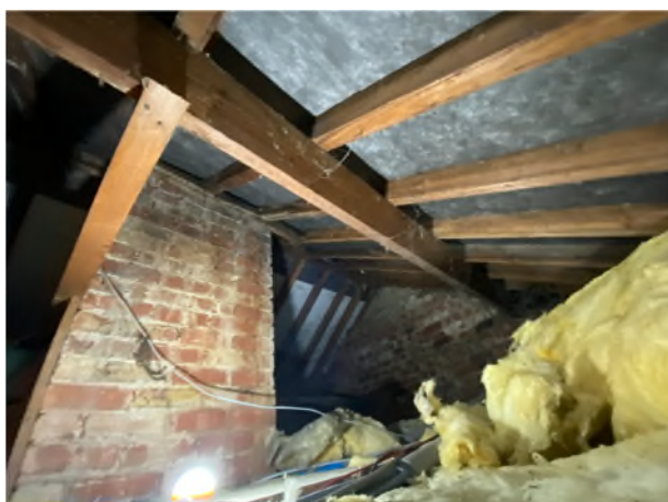
Figure 15: Fletton brick chimney and replacement roof structure in Phase 2
