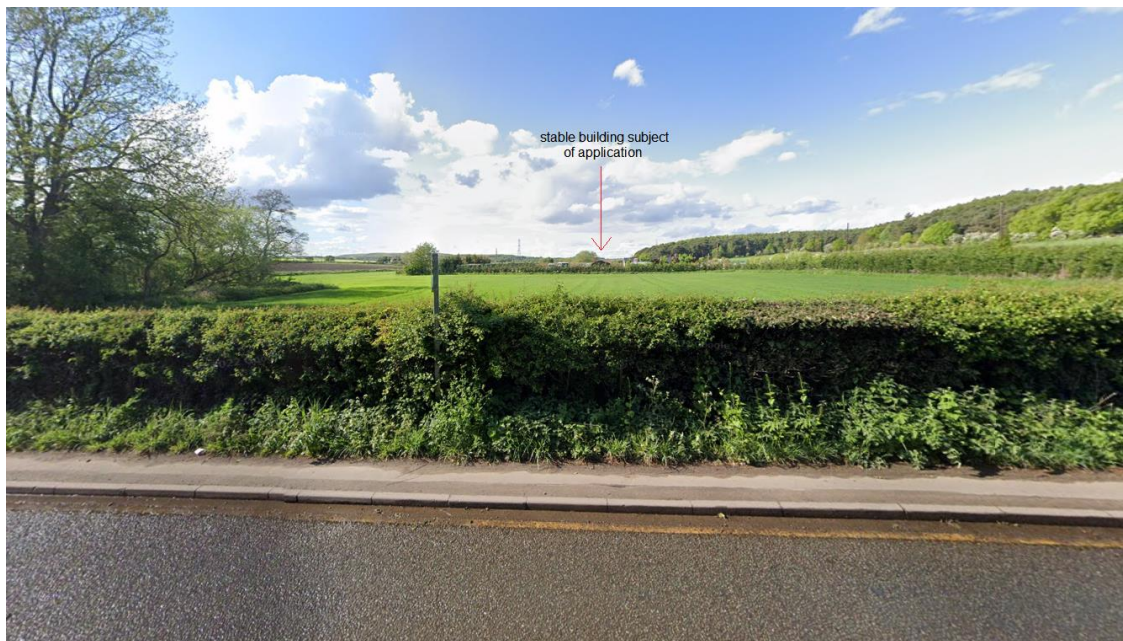
Figure 1: View of building from Rufford Lane
