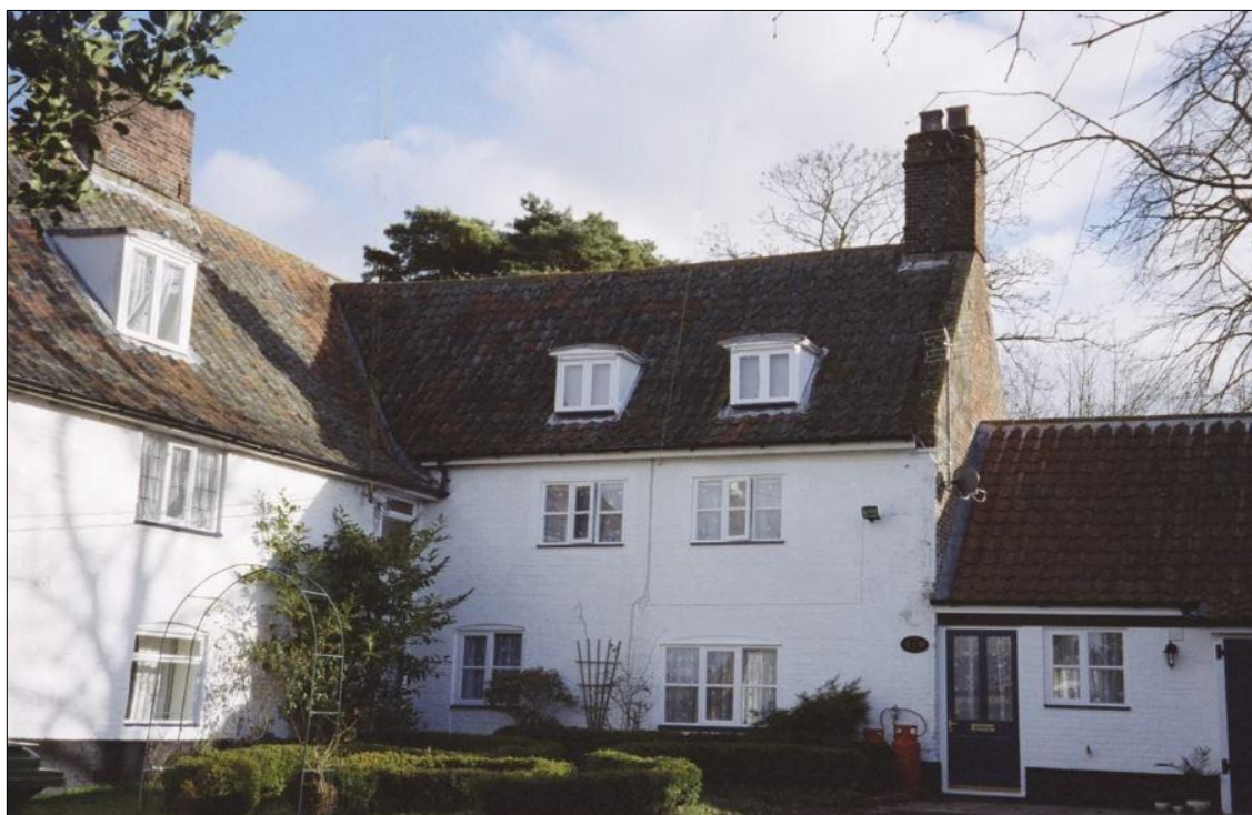
Existing West Elevation from Historic Archive
