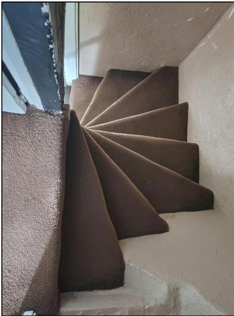
Existing Stairs which are difficult to navigate and dangerous to use.
