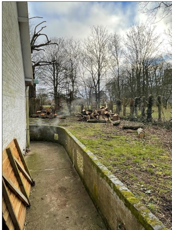
Existing Brick Retaining Wall to the South
