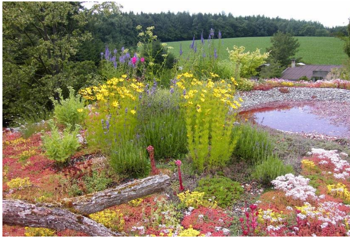
Figure 6: Example of dew pool on a green roof
