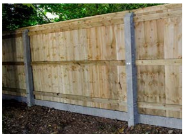
Proposed close board fencing to north boundary
