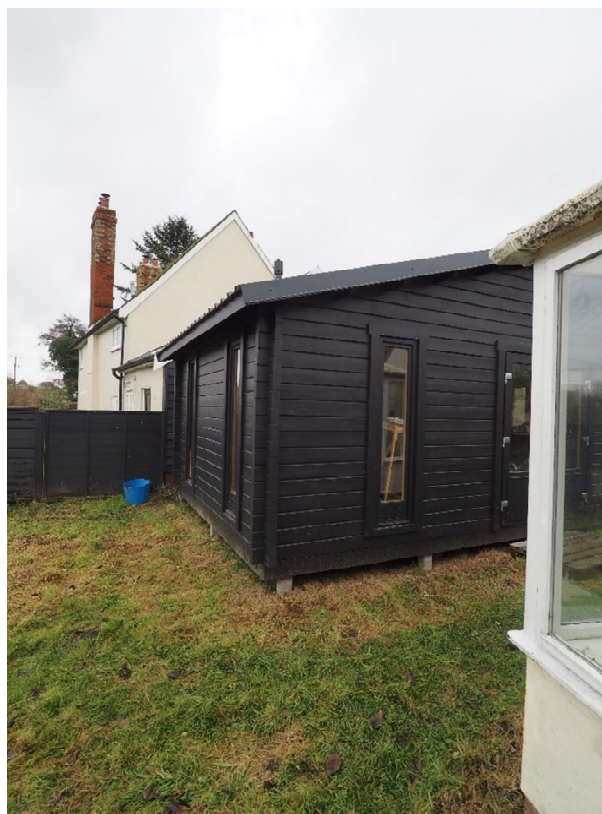
Figure 8: Looking at the new shed the curtilage of Claudes Cottage showing the concrete staddles it sits on.
