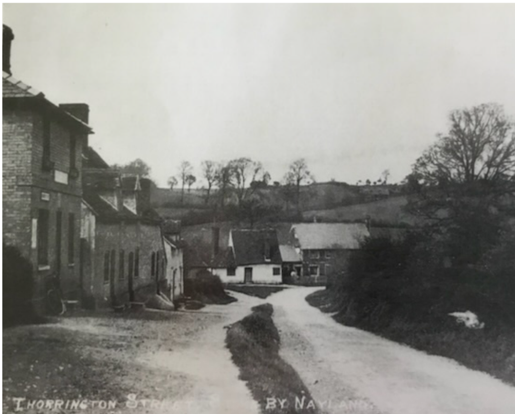
Figure 7: Looking North towards old bakery in what would become the curtilage of Claudes Cottage
