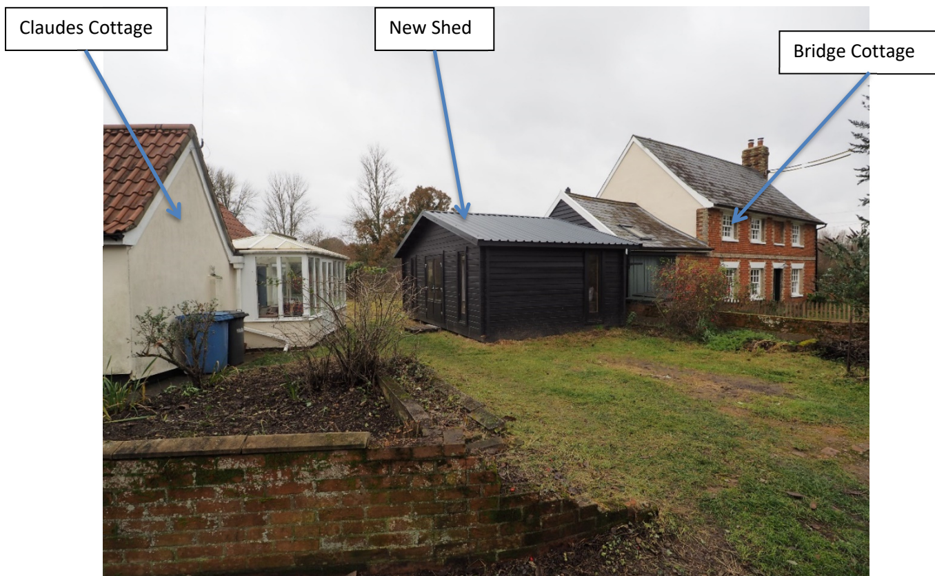
Figure 4: Looking North towards New shed in the curtilage of Claudes Cottage
