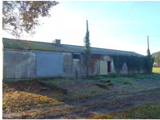
Photo 2: Stack of asbestos cement board in front of Structure 4
