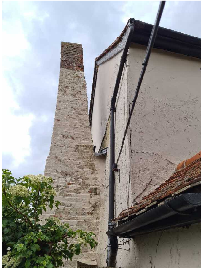
Fig 4: View of side elevation of rear chimney stack
