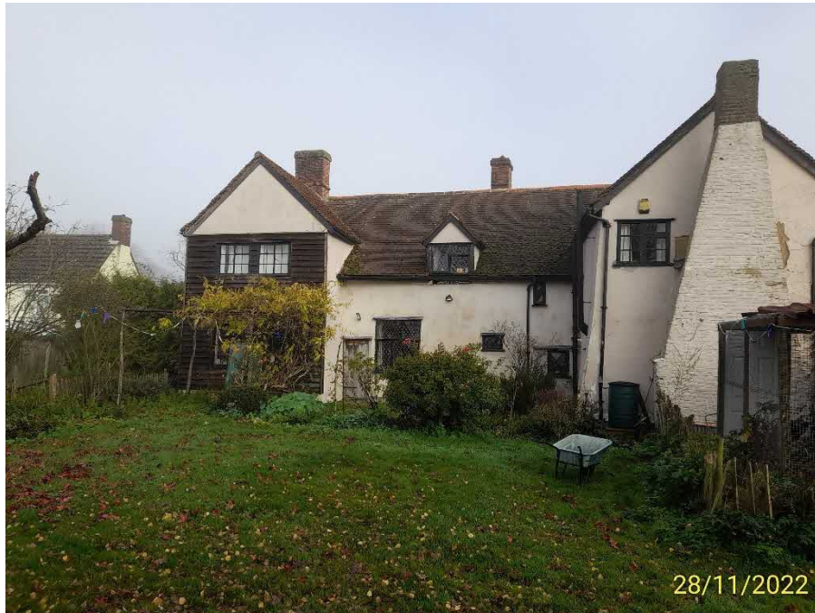
Fig 2: Rear (southwest) Elevation of Peverells with the chimney stack to the right
