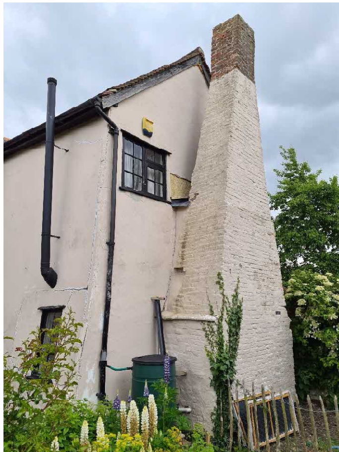
Fig 3: View of rear chimney stack
