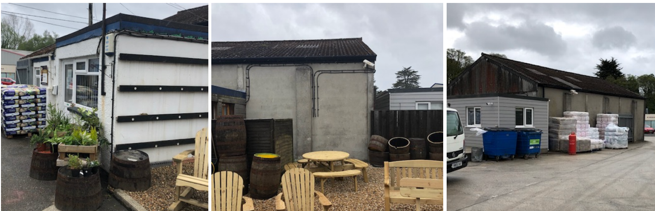
Buildings to be demolished
