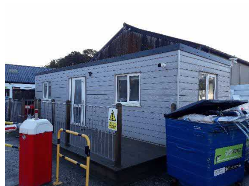
Figure 5 North side of Building 6
