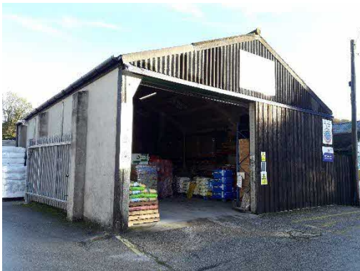
Figure 2 South side of Building 3
