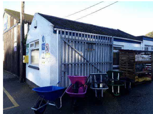
Figure 3 East side of Building 4
