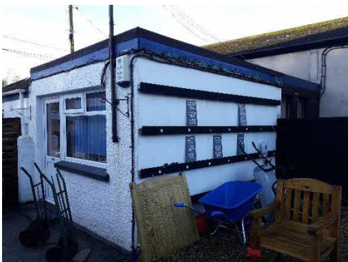
Figure 4 North side of Building 5
