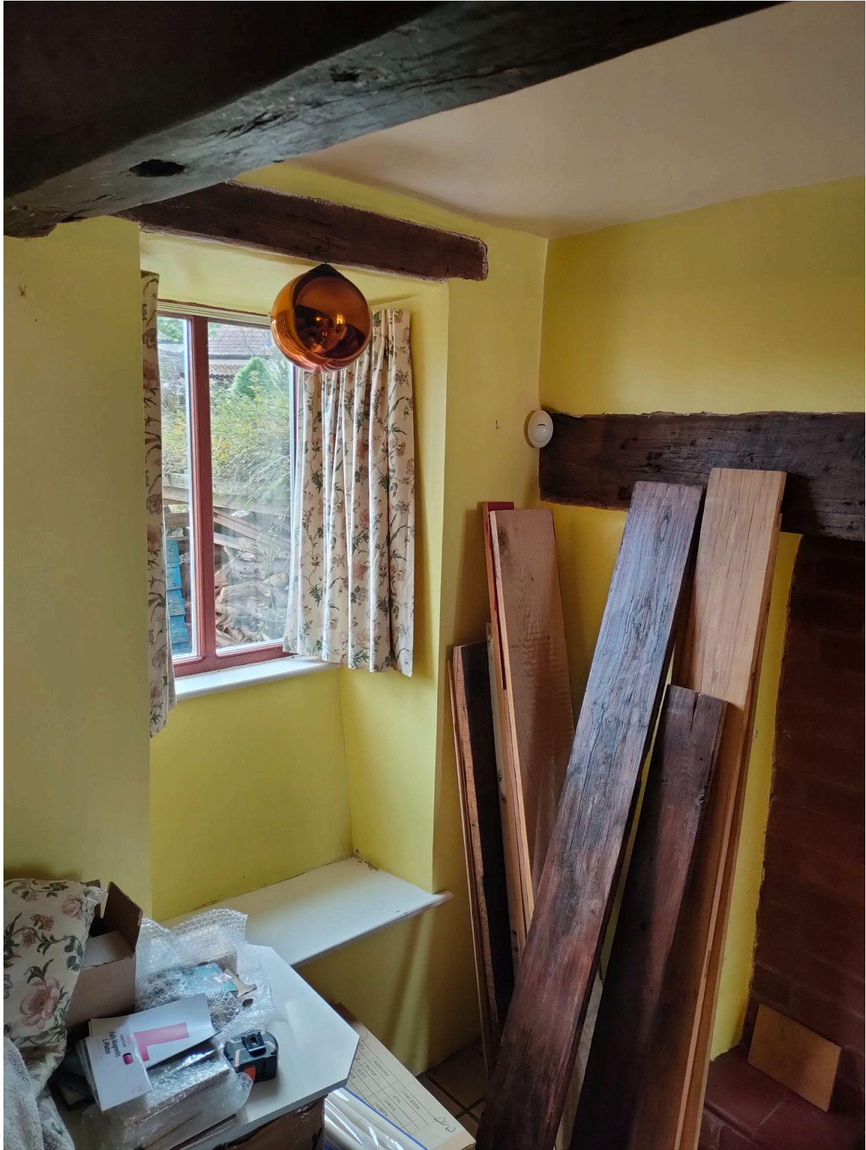
Window to garden - chimney
