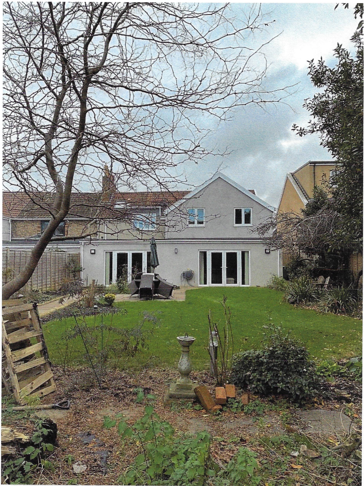
View from proposed Twin Unit looking back up to Main Dwelling.
