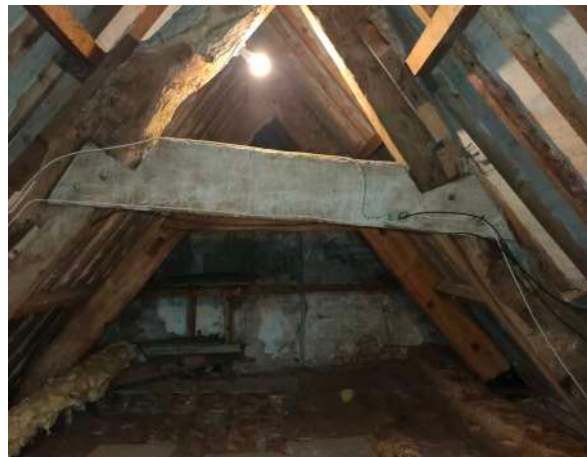
14. The main attic with historic principles and replacement common rafters
