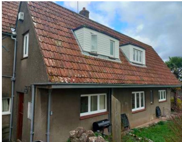
8. The rear extension
