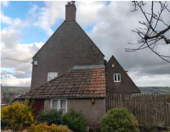
7. The southern gable end with rear extension
