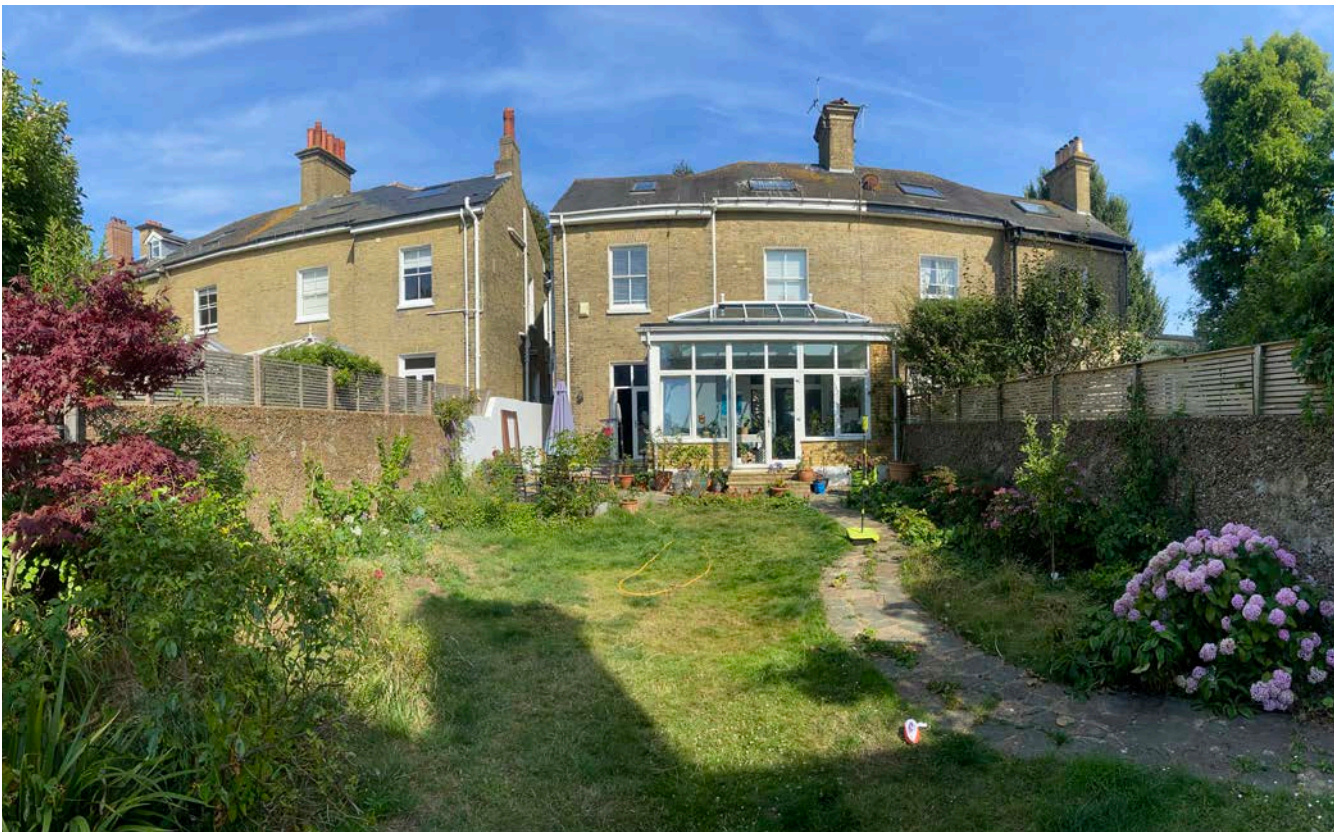
Above: Photo from the back of the rear garden looking east towards the rear elevation of 17 Denmark Villas.
