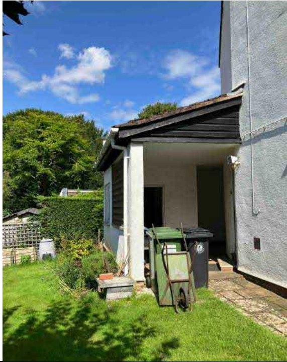
Covered walk through from southwest side
