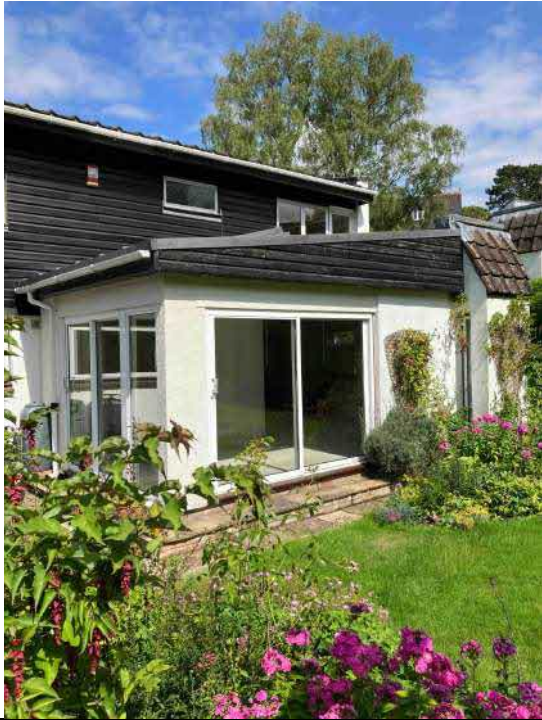
Southwest elevation glazed living room extension
