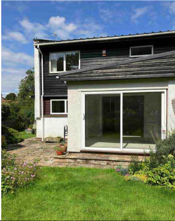
Southwest elevation LH side
