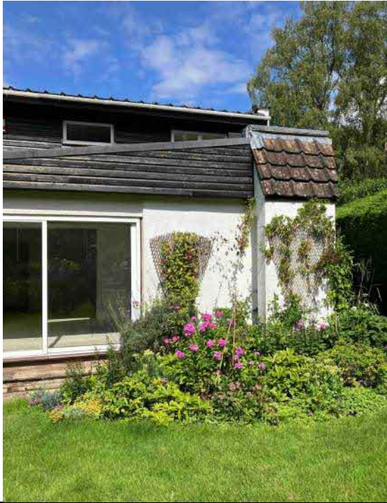
Southwest elevation RH side
