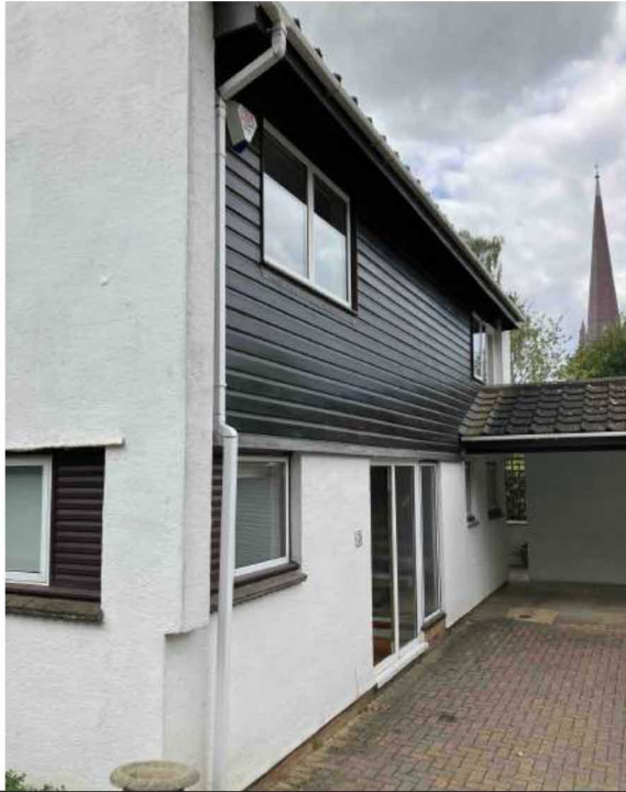
Northeast elevation showing the existing covered walk through
