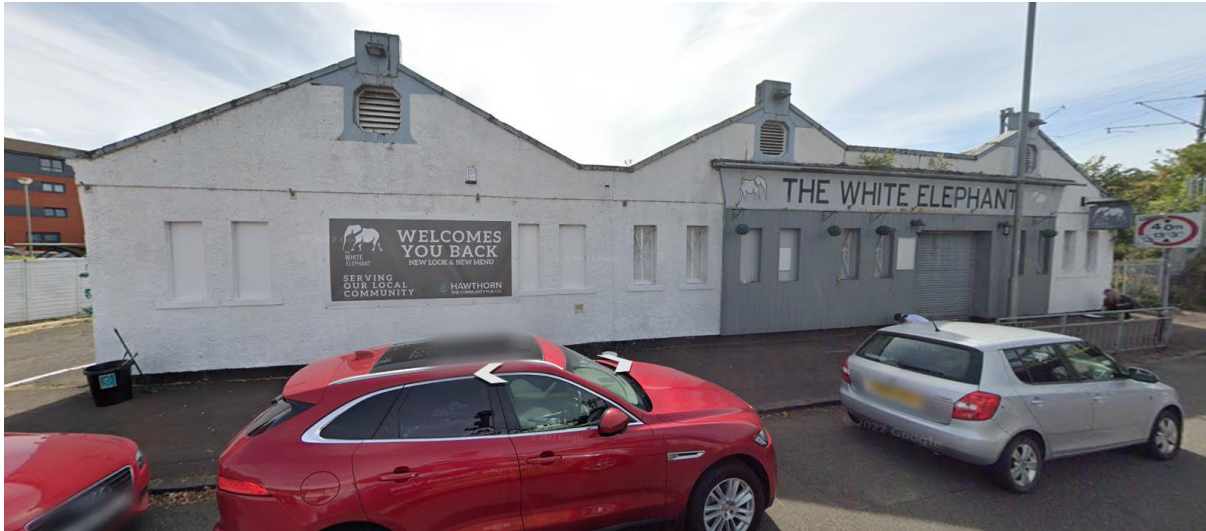
Fig 2: Street view of existing North Elevation from Merrylee Road.
