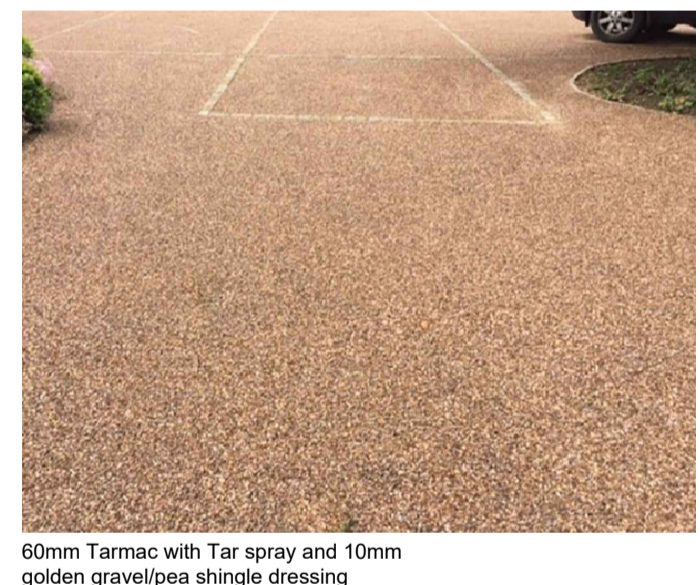
60mm Tarmac with Tar spray and 10mm golden gravel/pea shingle dressing
