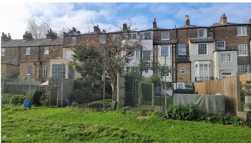
Figure 8: View of rear of terrace at southern end looking west showing a variety of rear extension designs
