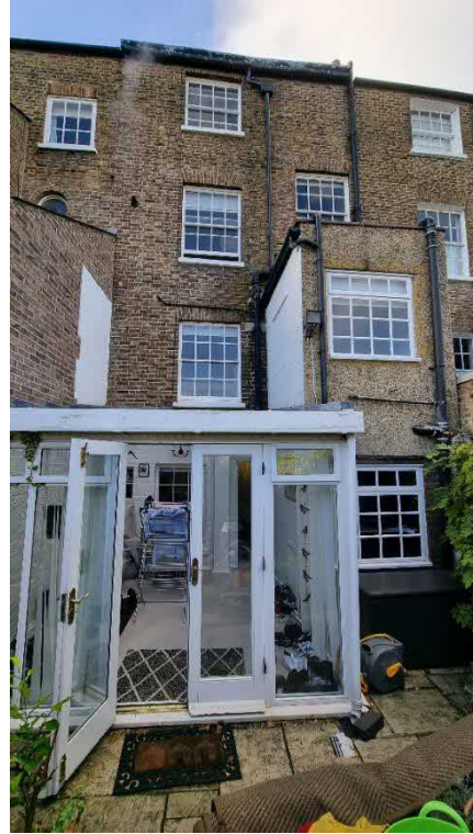
Figure 6: Rear elevation of application building at north end looking west
