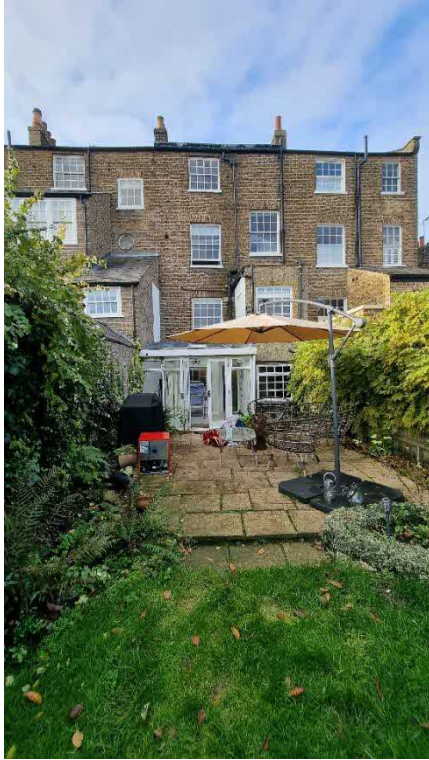
Figure 5: Rear elevation of terrace at north end looking west
