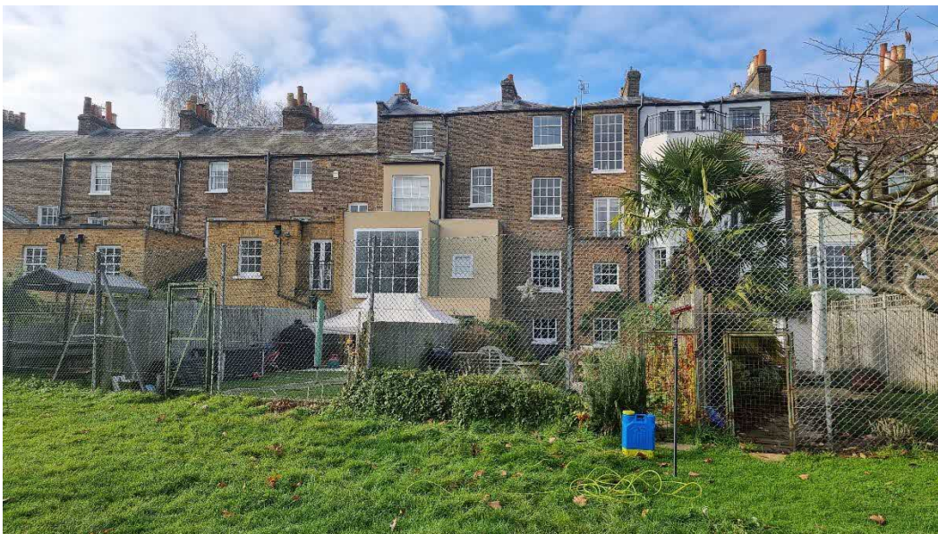
Images of the rear of the terraces.
