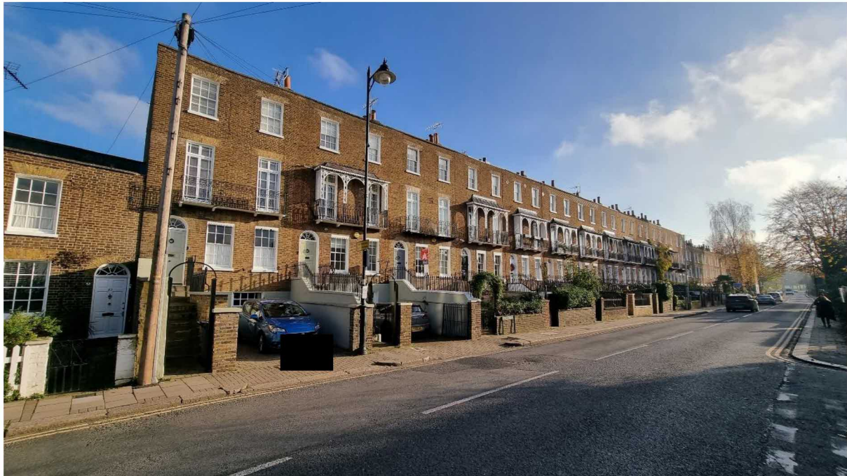
Front elevation of the terrace – application property 3 rd from the left.
