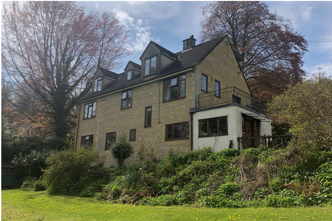
View of existing property from North
