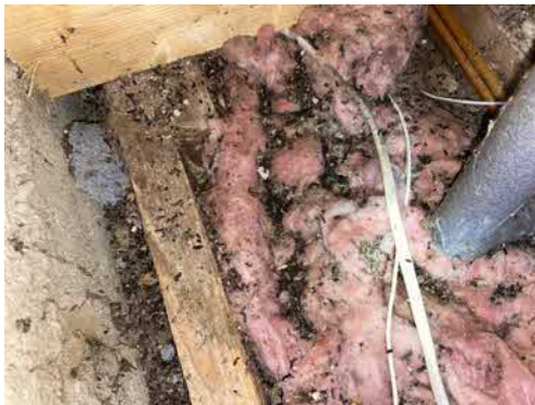
Photo 9: Bat dropping concentration within loft element. E1
