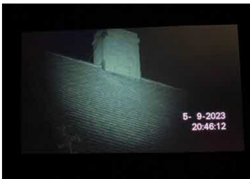
Photo 87: Example infrared camera view
