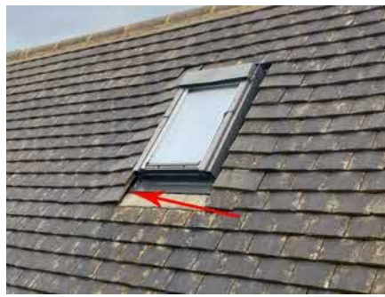
Photo 4: Red arrow points to raises surrounding skylight. E2.
