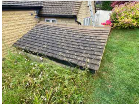
Photo 14: Concrete tiles cladding roof of E3.
