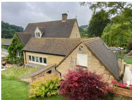
Photo 3: E2 – east-facing elevation showing external timber doorway to loft void.
