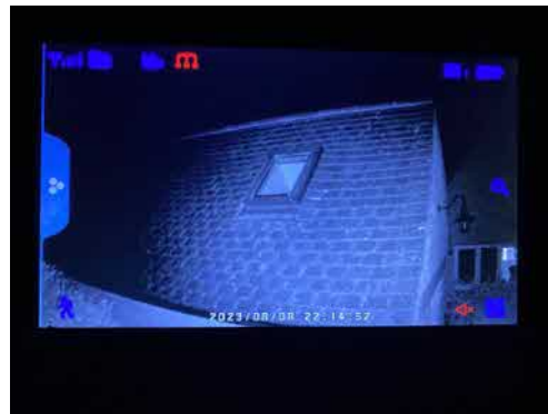
Photo 16: Example infrared camera view
