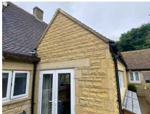
Photo 6: Stonework of gable end. E2.
