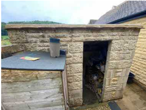
Photo 73: E3 - Block-built storage shed
