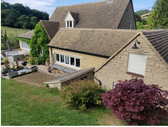
West elevation - Existing rear extension
