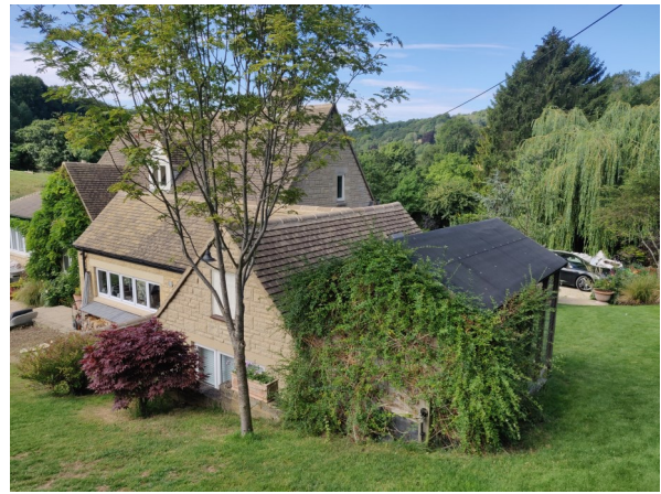
North west elevation - Existing rear extension
