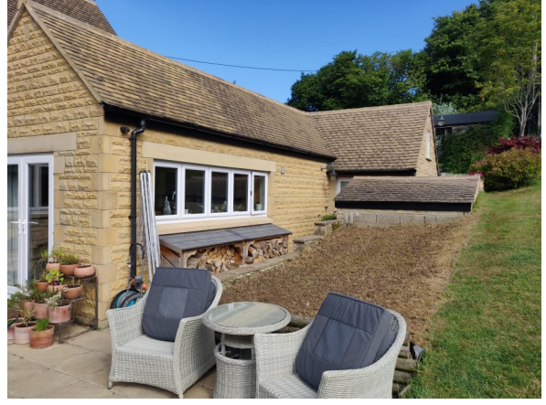
West elevation - Existing rear extension
