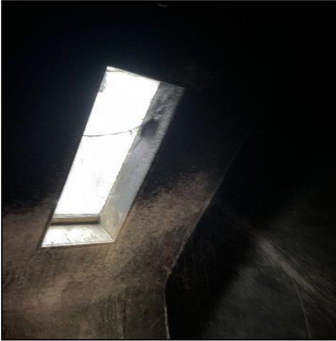
P 3: First Floor – areas of smoke damage (Sedgwick 2024)
