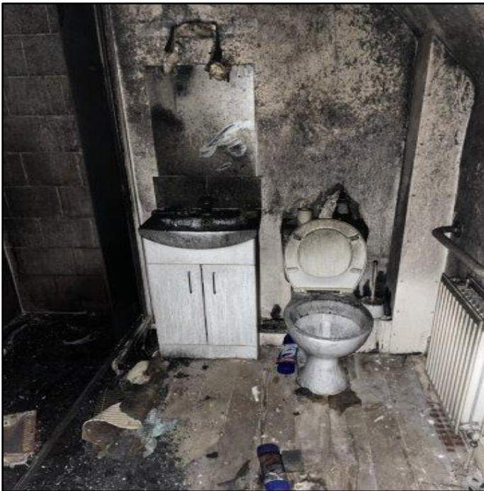
P 4: First Floor – areas of smoke damage (Sedgwick 2024)
