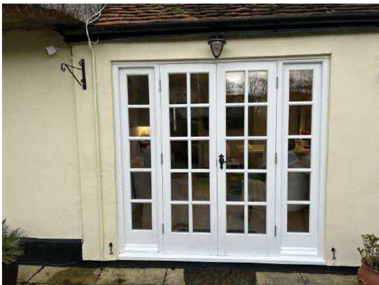
Photograph of the existing patio door to the kitchen to be replicated to the back of the new dining area.
