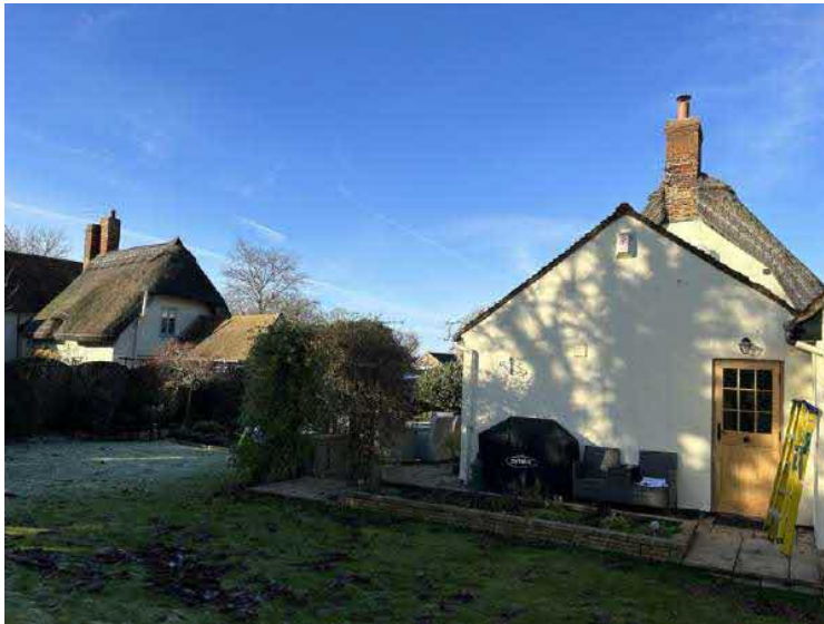
Photograph of the rear of the kitchen where the extension is to extend out in the same line and roof pitch.
