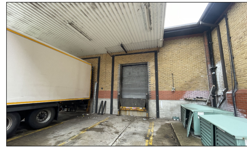
EXISTING UNLOADING BAY AREA PHOTOGRAPHS
