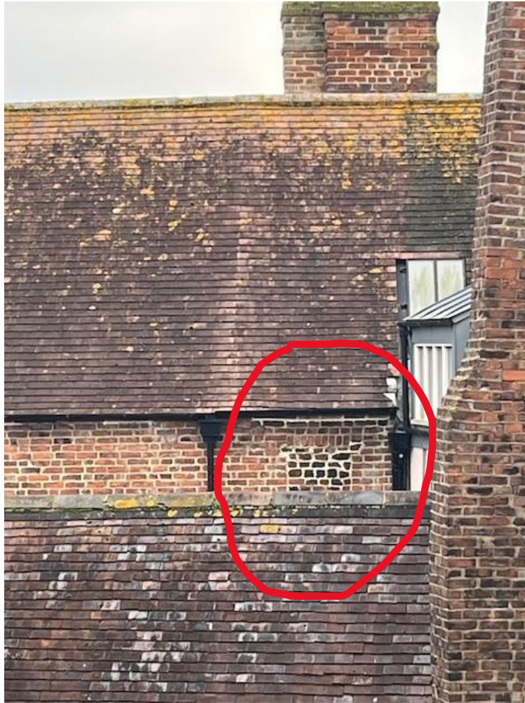
External view of Structural opening of existing historic window
