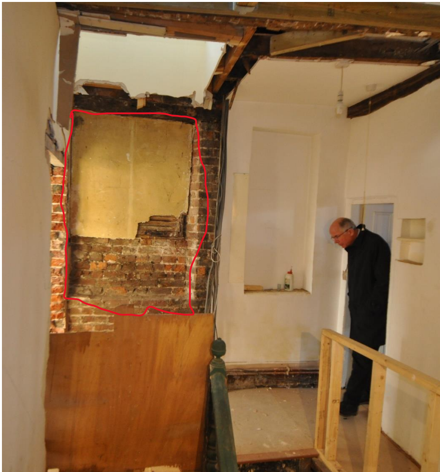
Structural opening of existing historic window from within the staircase
