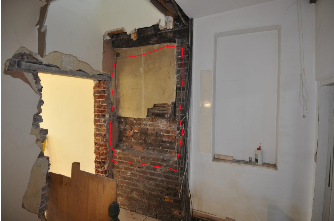
Structural opening of existing historic window from inside
