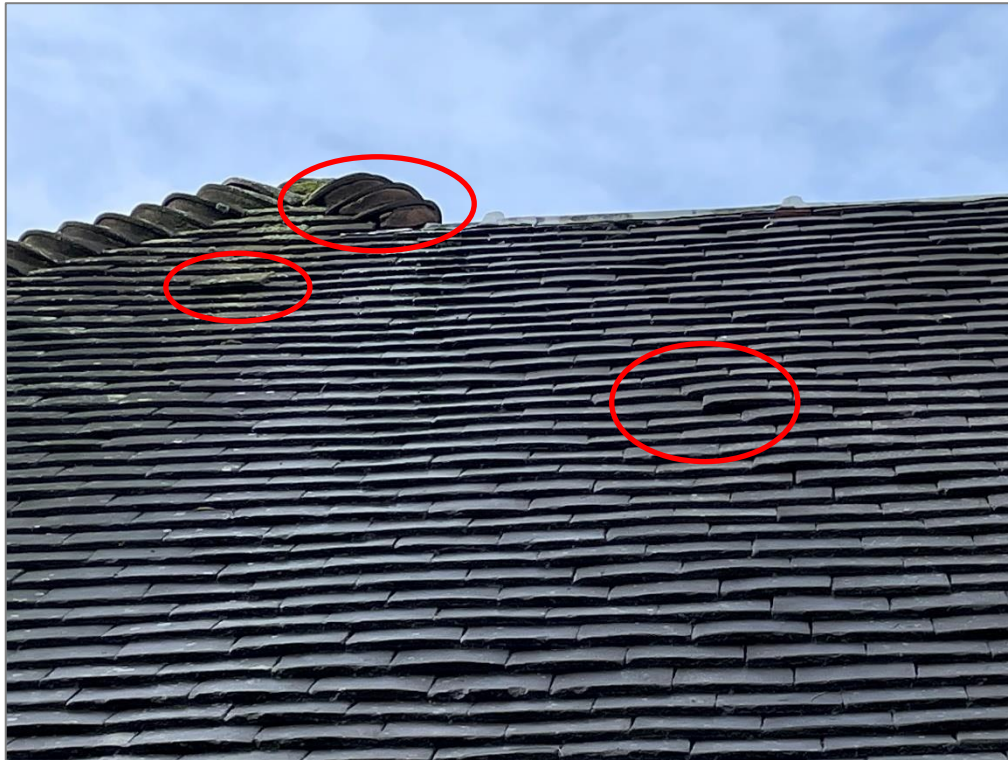
Photograph 3: Example of gaps under roof and ridge tiles (circled red) that could provide bat access.
