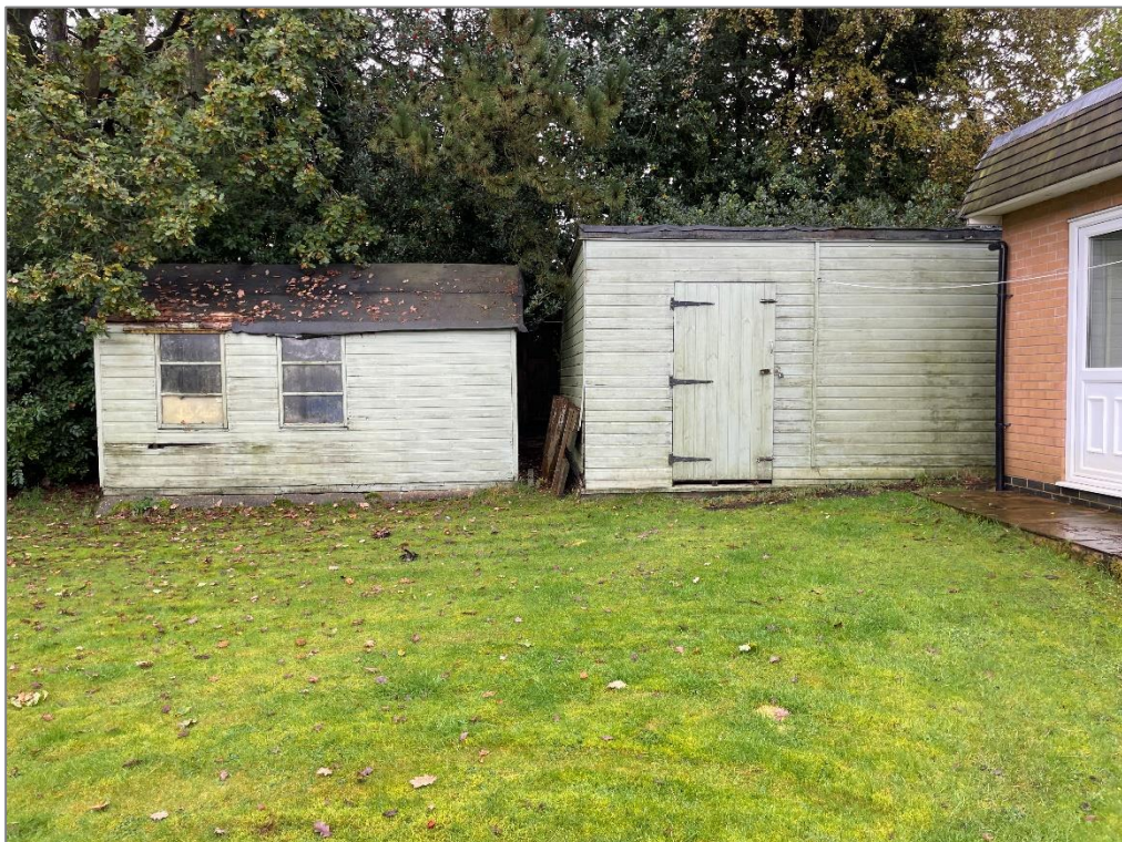
Photograph 7: Wooden garden sheds (Buildings 2 and 3).
