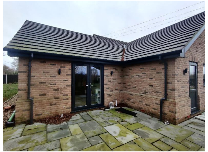
Photo 2 Southeast corner of the dwelling, where the new rear extension is proposed
