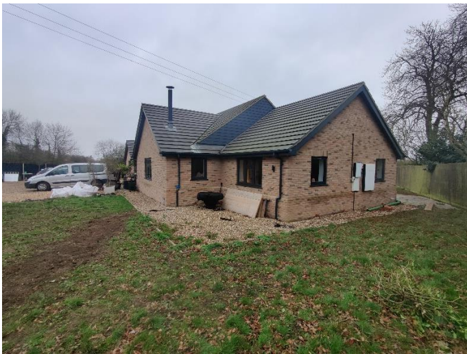
Photo 3 Southwest corner of the dwelling, where the new rear extension is proposed
