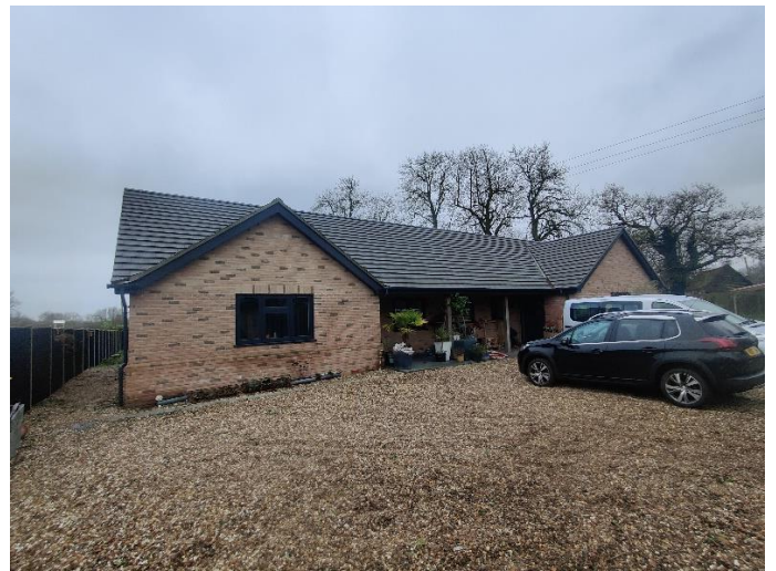
Photo 4 West elevation of the dwelling and adjacent gravel driveway
