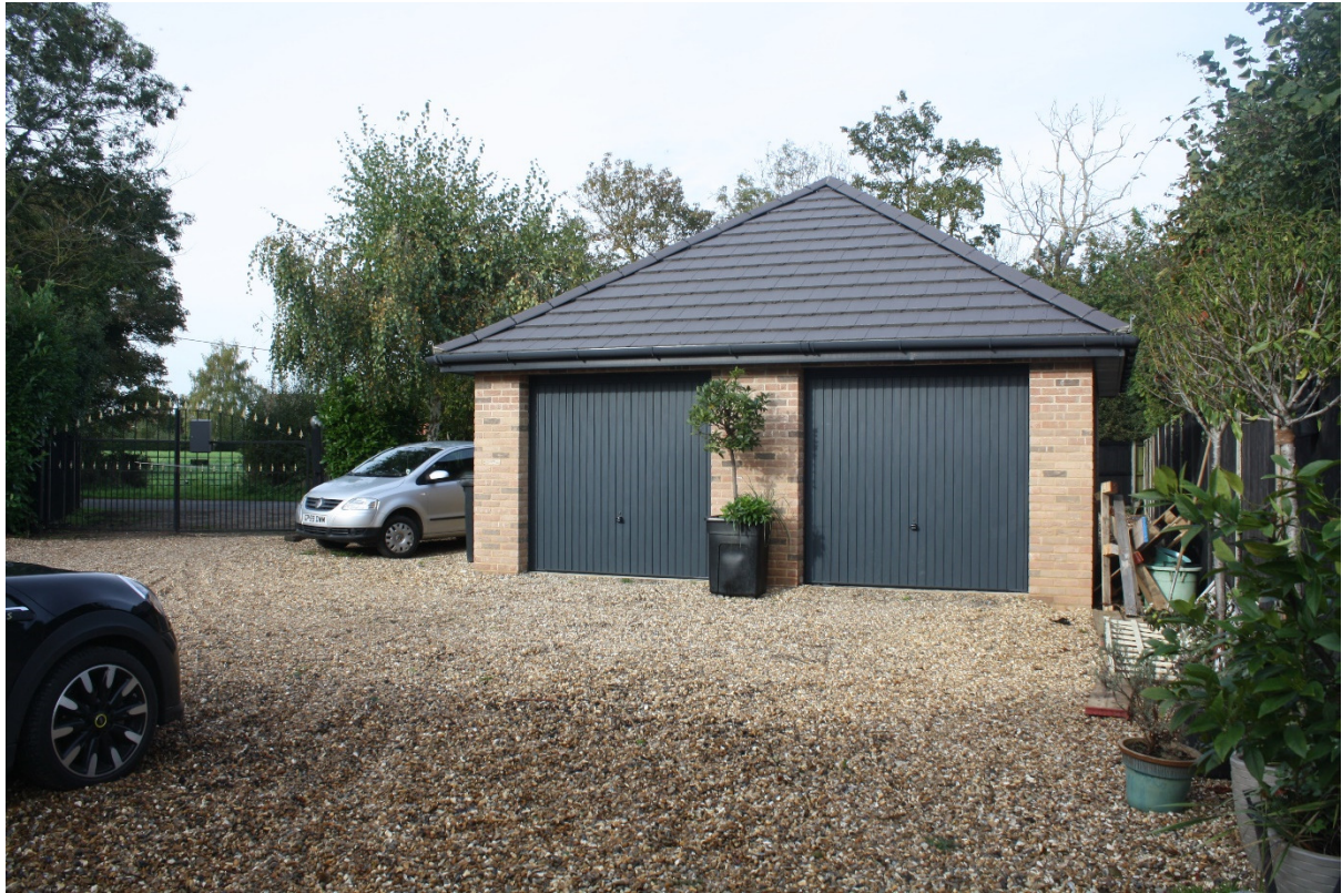
Photo 3 - Double garage (northern corner of site)
