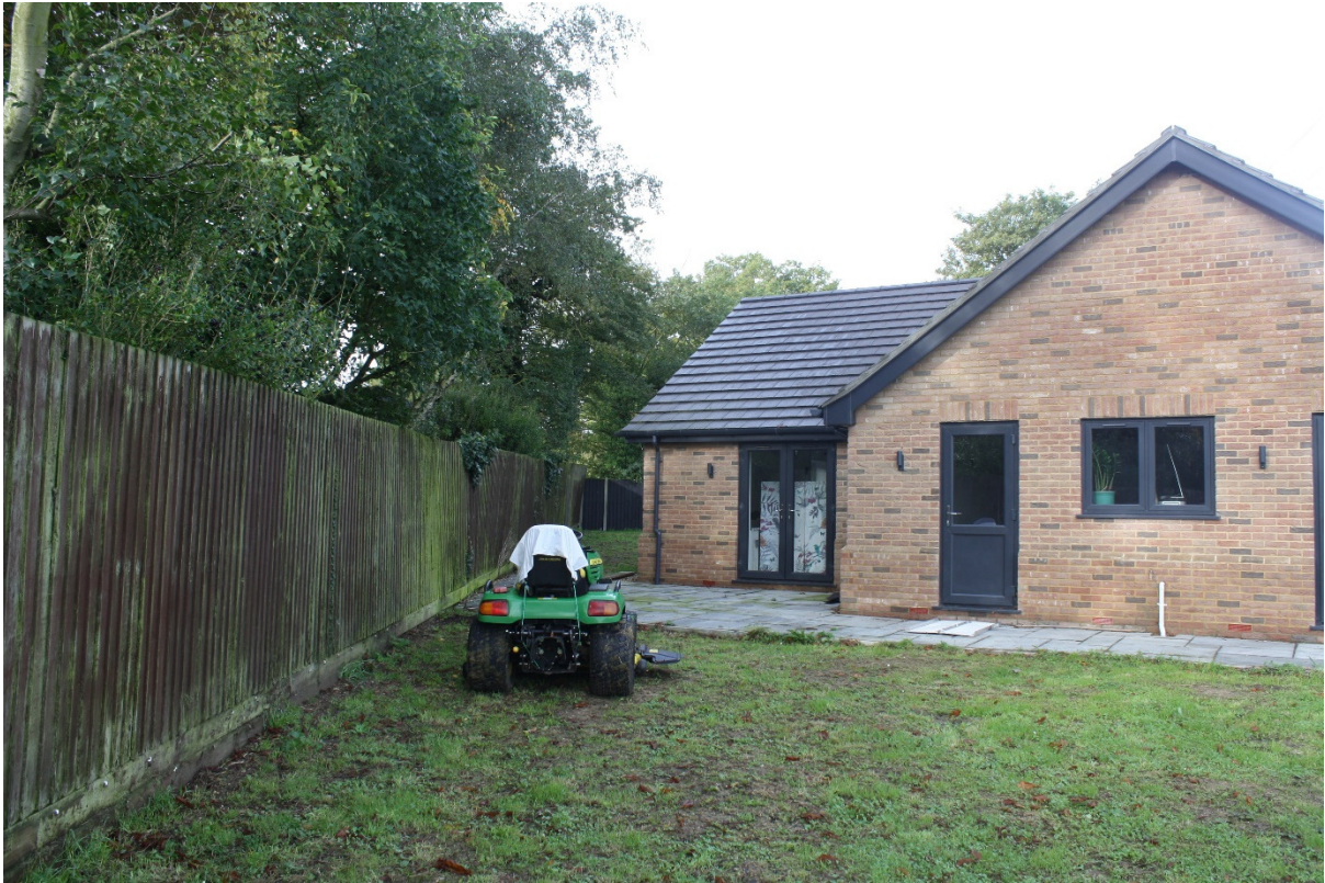
Photo 5 - Rear elevation and patio (proposed rear extension)
