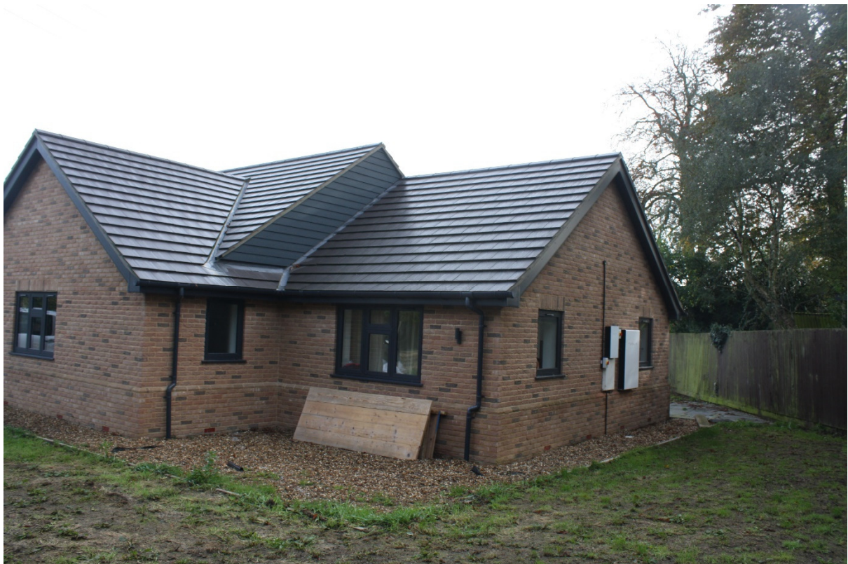
Photo 4 - Side (West/South) Elevation
