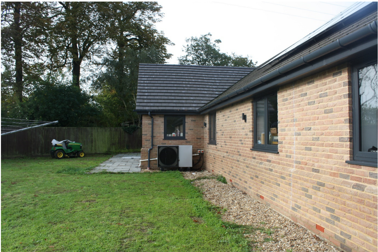
Photo 6 - Rear elevation and patio (proposed rear extension)
