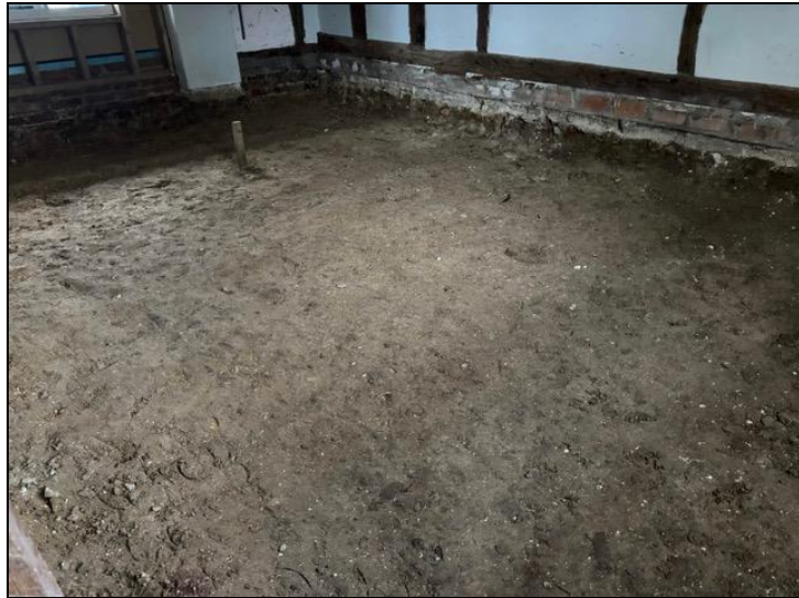
Internal shallow floor lowering
