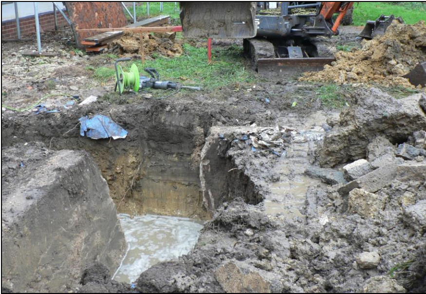
Trench at west end
