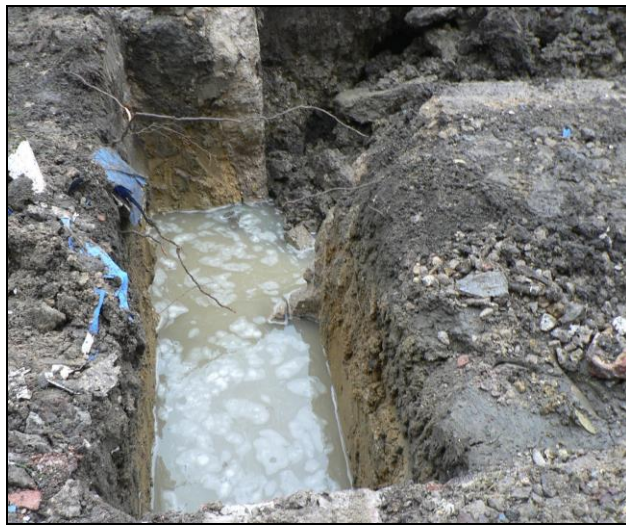
Foundation trench at eastern end
