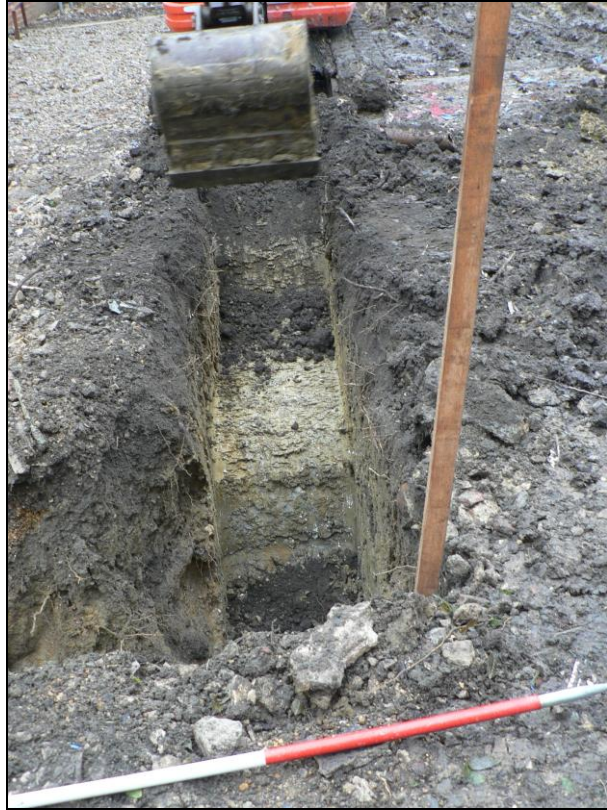
Excavation of foundation trench
