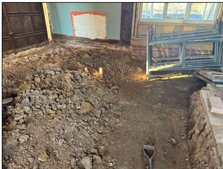
Internal floor lowering
