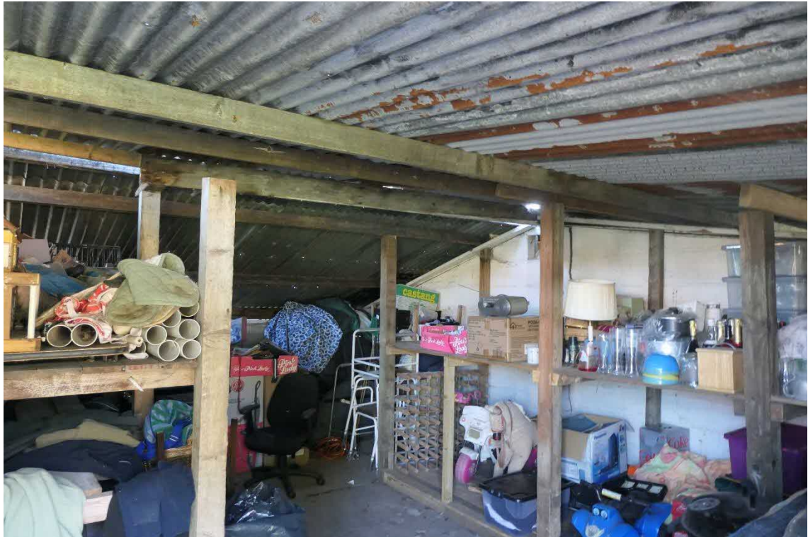
Photo 6, internal view of a compartment within building one, looking south.
