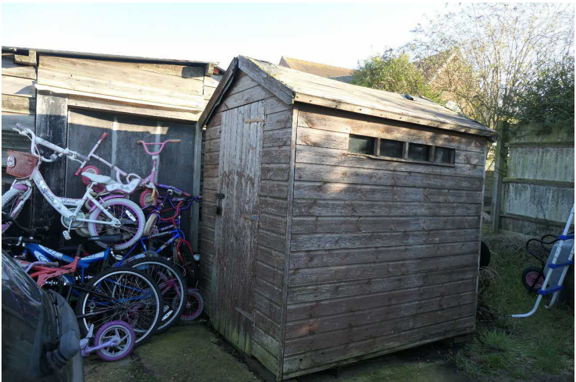
Photo 9, northwest and southwest aspects of building four.
