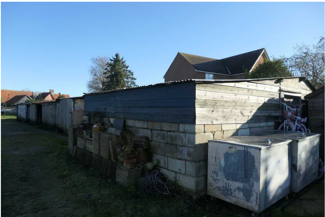
Photo 5, southwest and northwest aspects of building one.
