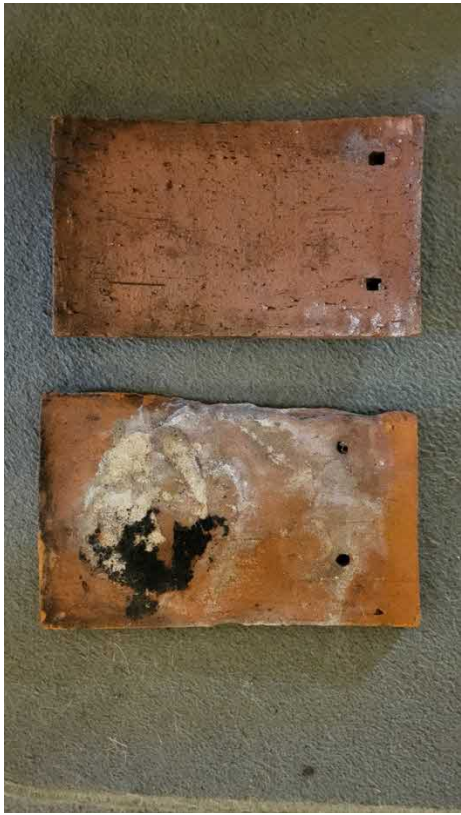
Roof tiles rear face
