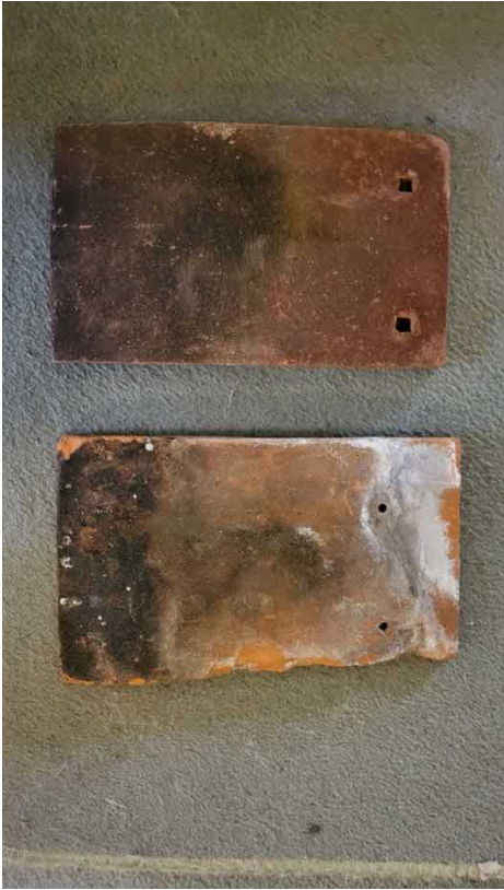
Roof tiles front face
