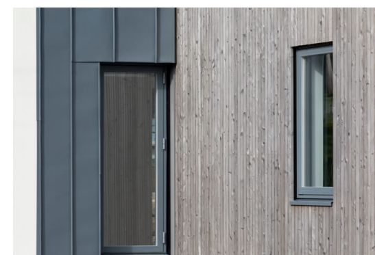
Larch cladding- left to weather to natural grey Anthracite grey windows, fascias and bargeboards etc.
