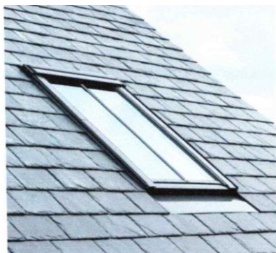
Typical conservation rooflight.
