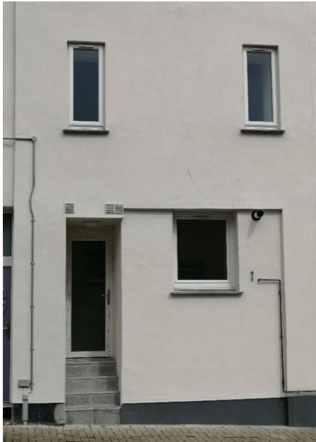
West elevation showing 3 single pane double glazed UPVC windows
