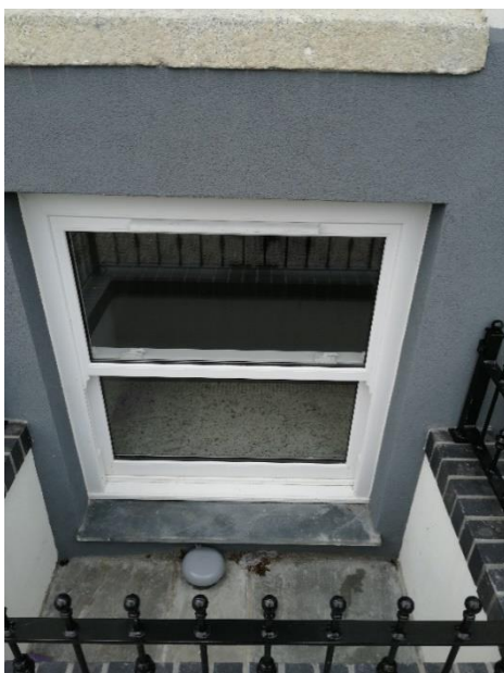
South elevation showing basement UPVC double glazed windows.
