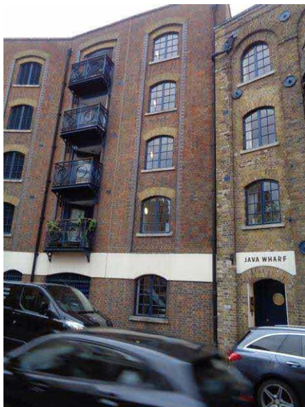
Front of property.
