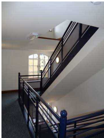
Staircase within building.
