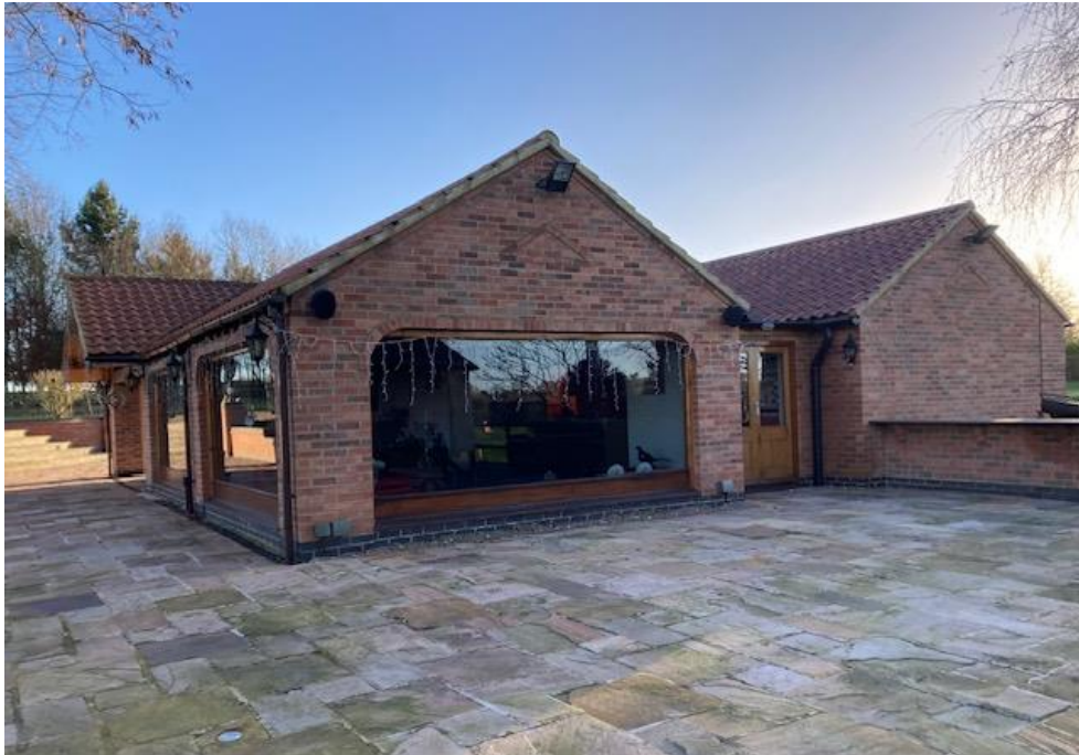
10. The rear north west elevation of Car Hill Grange and stone paved areas.
