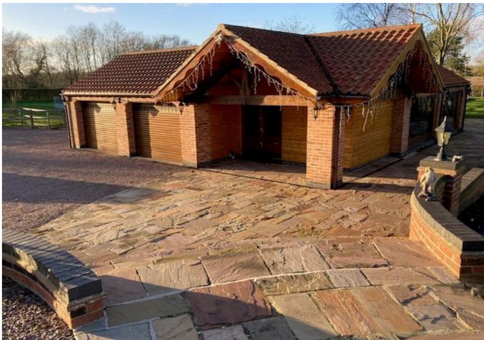
5. Looking north west across the top step.
