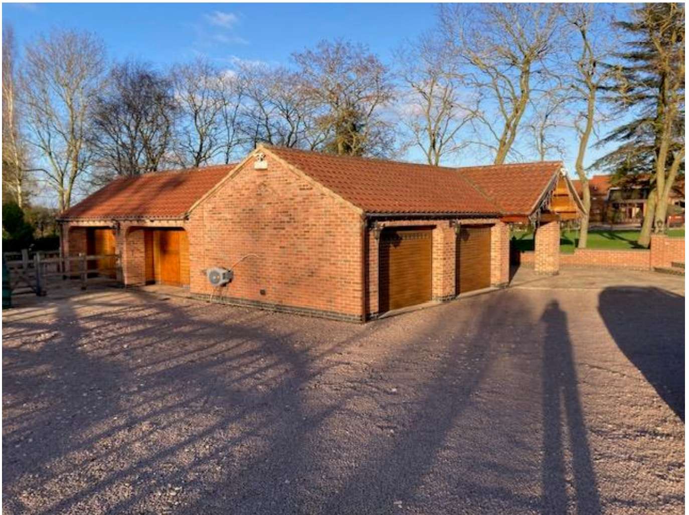
1. The front south corner of Car Hill Grange – front stone chipping surfaced car turning and parking area.
