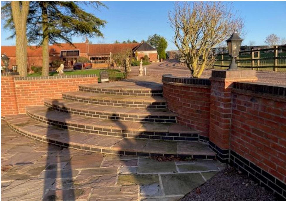
4. Steps at the front south east corner between brick boundary walls.
