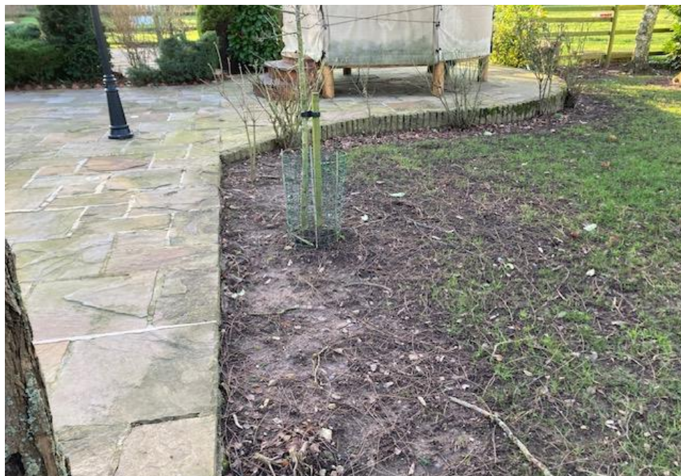
9. The rear north edge of the stone paving.
