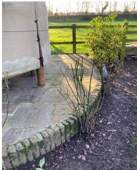
11. The rear curve edged stone slab paving and brick kerb.
