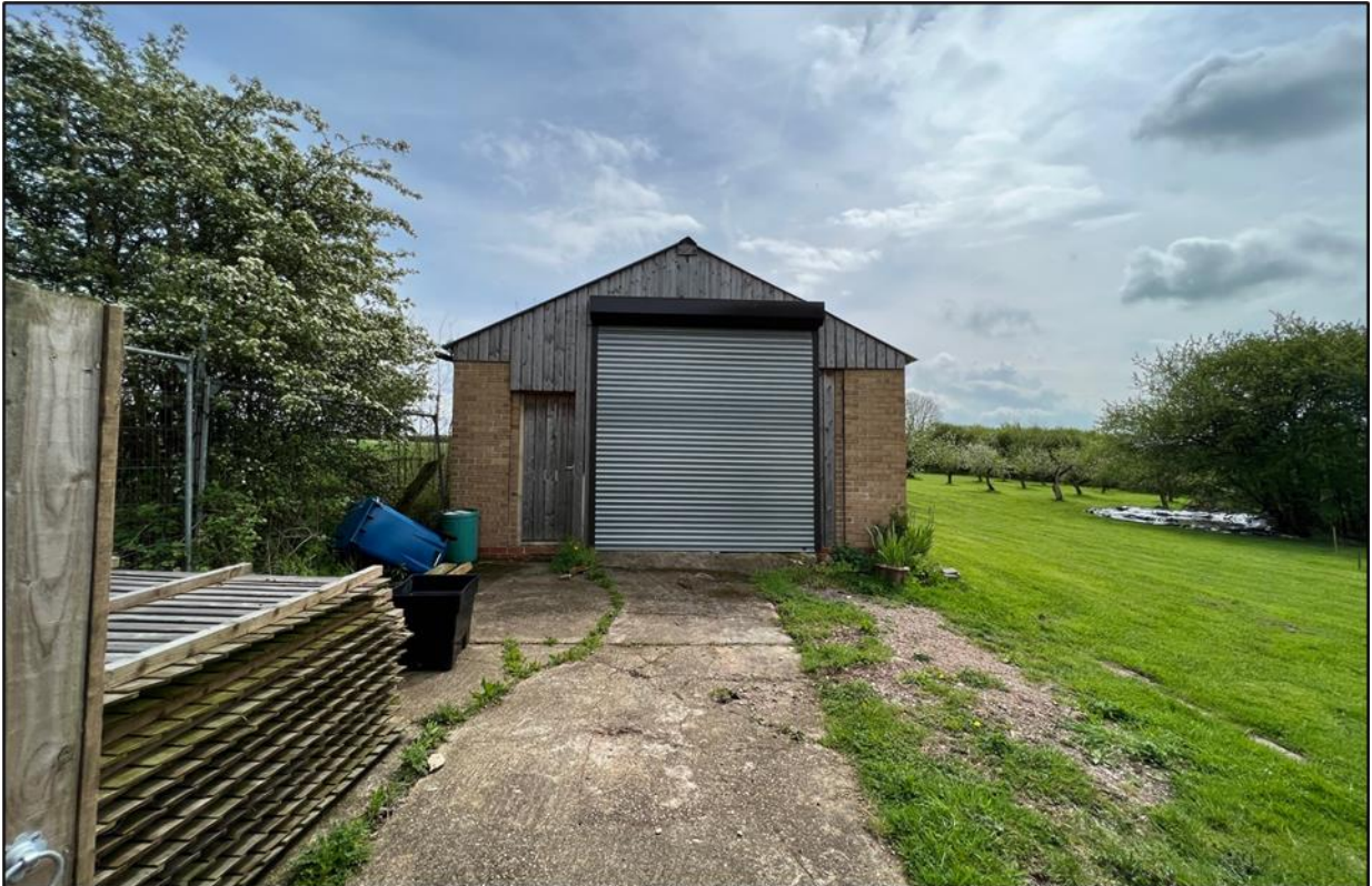
Photograph 3 – Large brick-built shed with sloped corrugated metal roof covering to the east of the main dwelling, taken from the north west. This building is outside of the proposed works.
