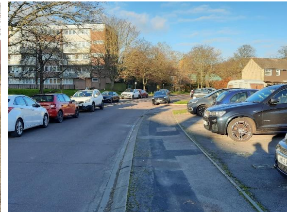
Photo 4: Timsbury Drive facing north. Road-side parking bays both sides.
