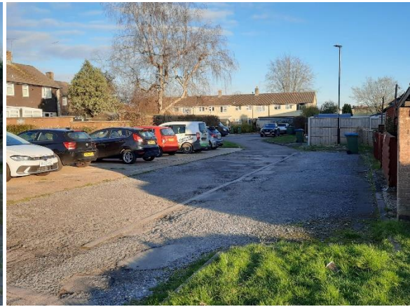
Photo 2: Second Lockerley Crescent off-road Parking area, facing east.
