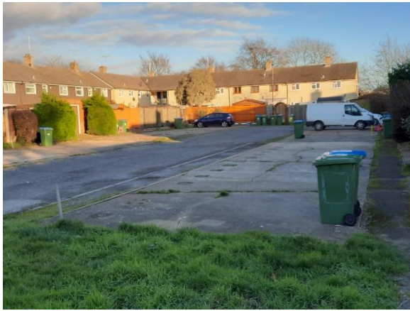
Photo 1: Lockerley Crescent off-road parking. Facing east.
