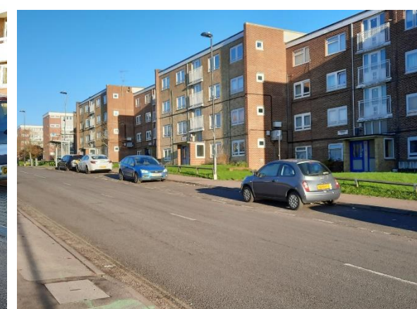
Photo 6: Wimpson Lane. Road-side parking bays. Facing north.
