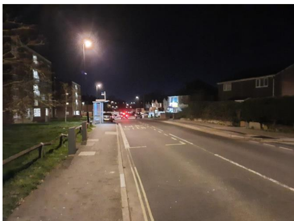
Photo: 21: Wimpson Lane facing south
