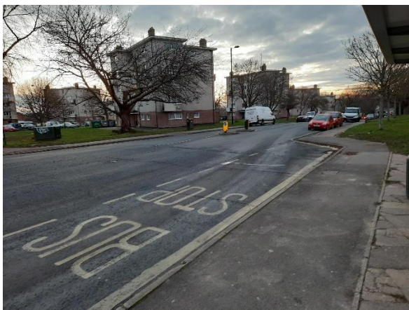
Photo 11: Redbridge Hill, facing west.
