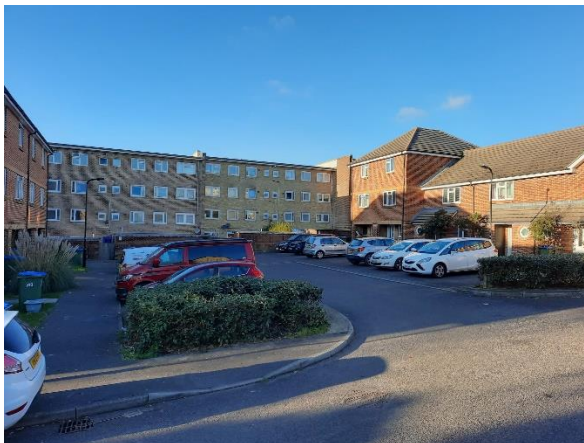
Photo 9: Western end of Irving Road.
