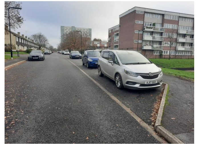
Image 3: Irving Road (leading east). Parallel parking spaces exist with kerbs set back and vehicles adjacent to the two road lanes.
