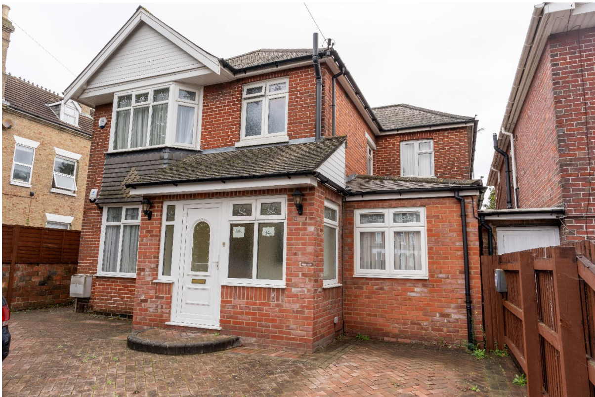
Figure 1: Front (south-west) elevation of 34a Westridge Road.
