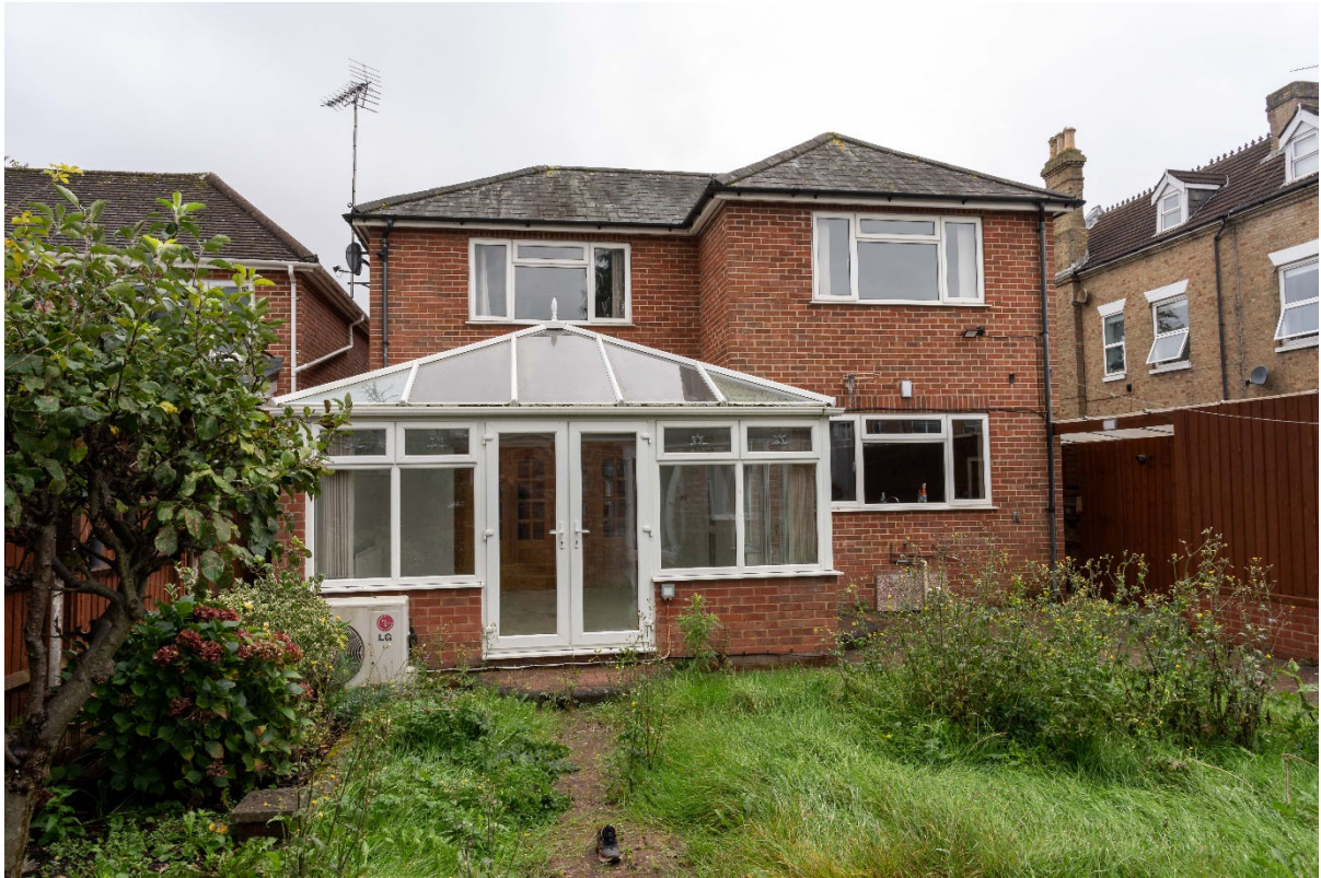
Figure 2: Rear (north-east) elevation of 34a Westridge Road.
