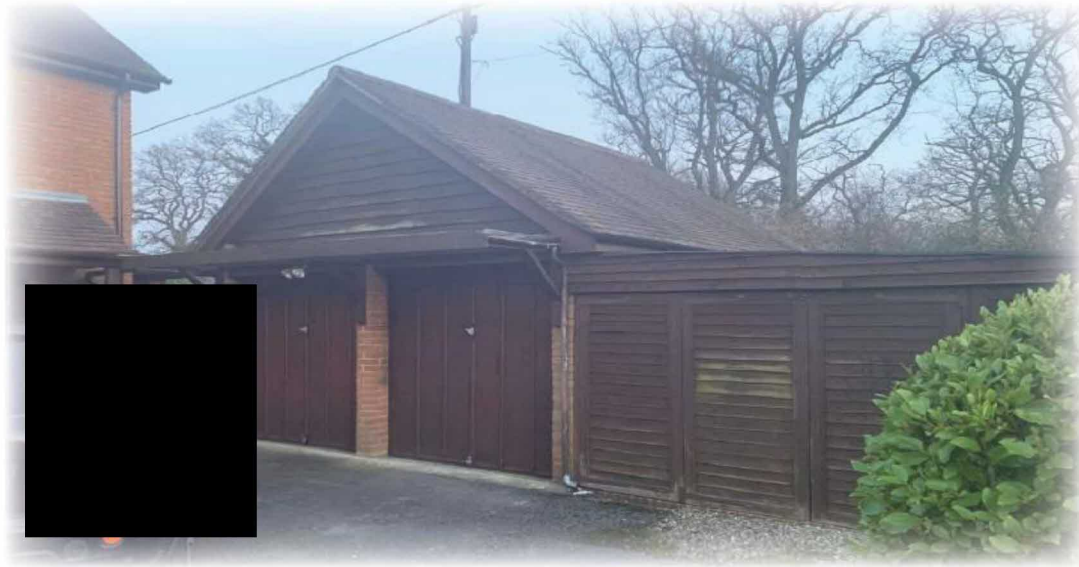
Above: Existing detached two double car garage for four cars
