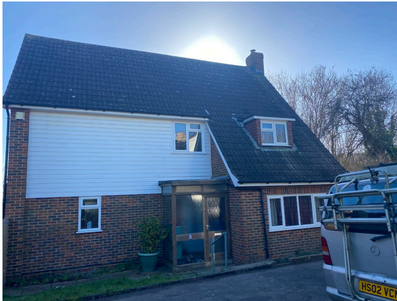
Front view from front driveway
