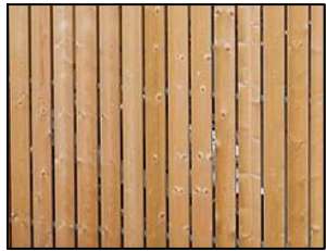
02 & 03 Vertical timber cladding
