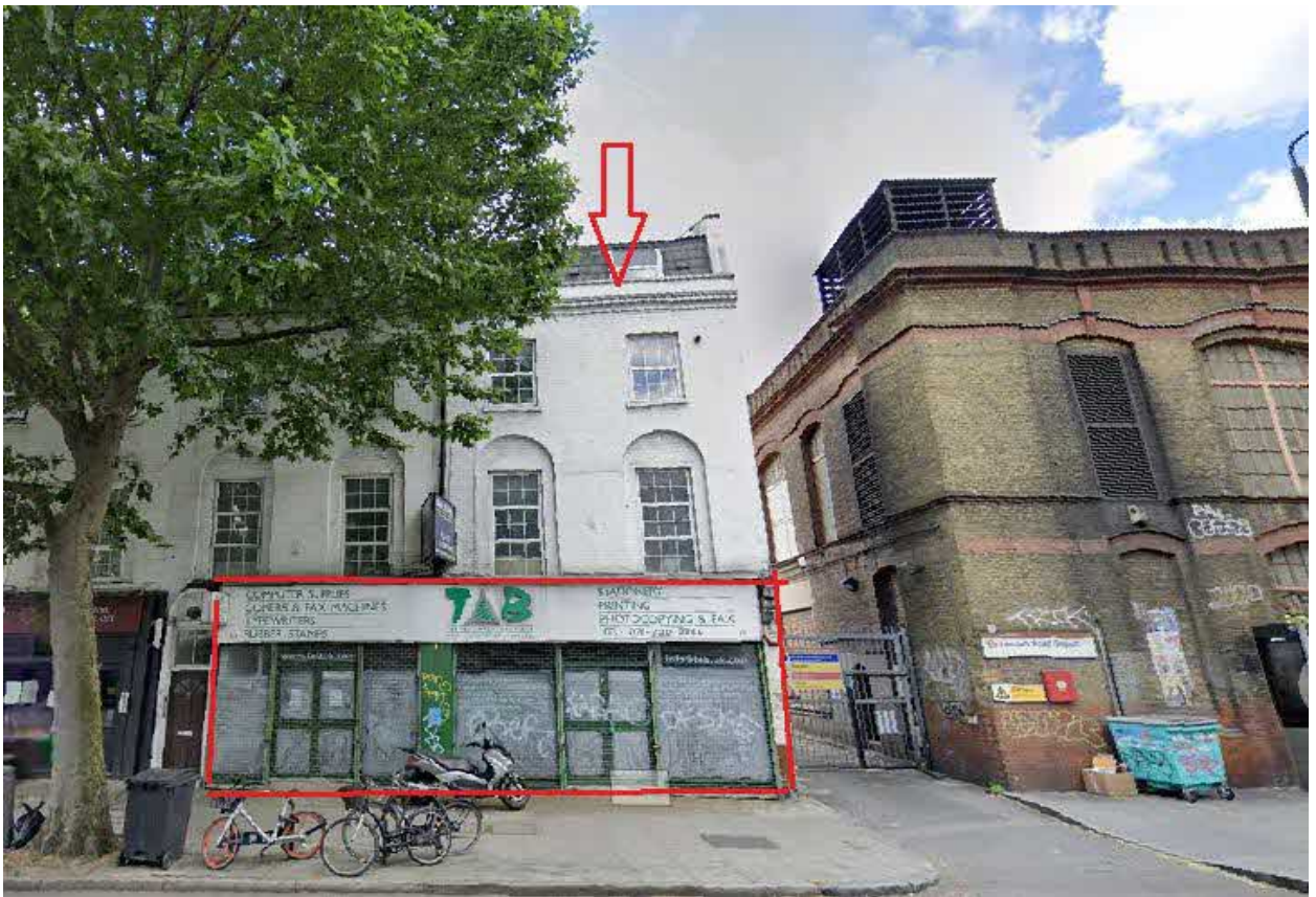
The highlighted portion on photo shows the site of the development. Page 4 of 17
