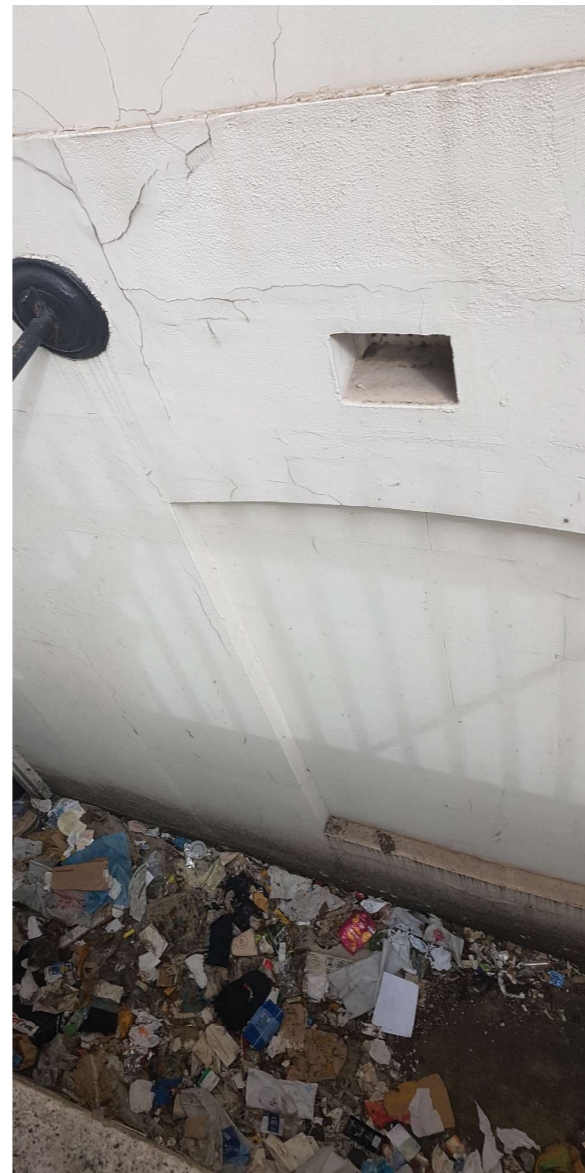
Arch 01 looking down through lightwell
