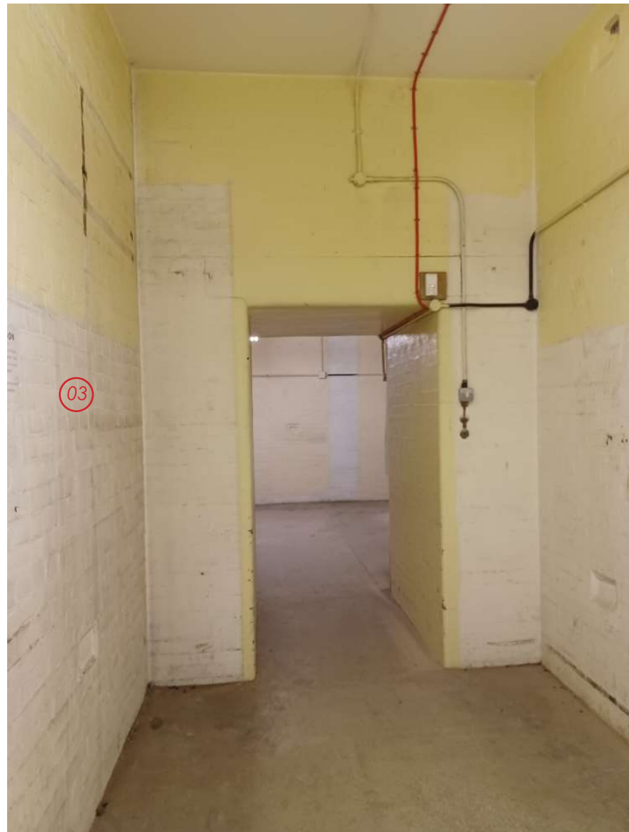
Bank vaults showing no apertures visible internally behind the masonry vault lining walls
