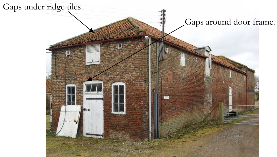
Figure 1 – Barn 1, south elevation.
